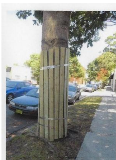
Figure 1. Indicative Trunk Protection
