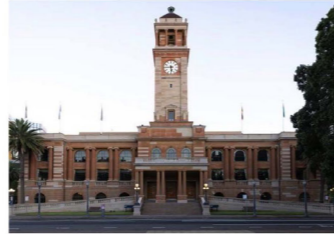
EXISTING CITY HALL 290 KING STREET NEWCASTLE
