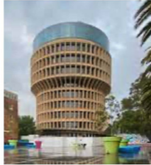
EXISTING KINGSLEY HOTEL 282 KING STREET NEWCASTLE
