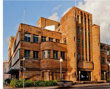
EXISTING NESCA HOUSE 300 KING STREET NEWCASTLE
