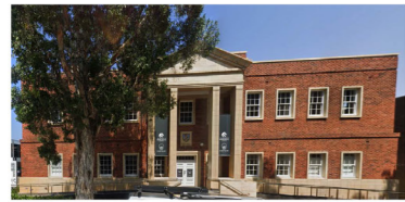
EXISTING NORTHUMBERLAND HOUSE 20 AUCKLAND STREET NEWCASTLE
