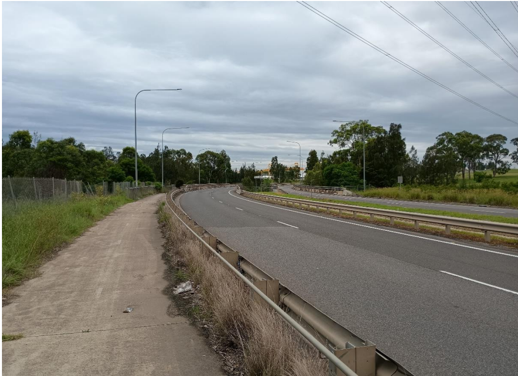
Photograph 11: Lenore Road at Service Alignment Chainage CH 1700 m Facing East
