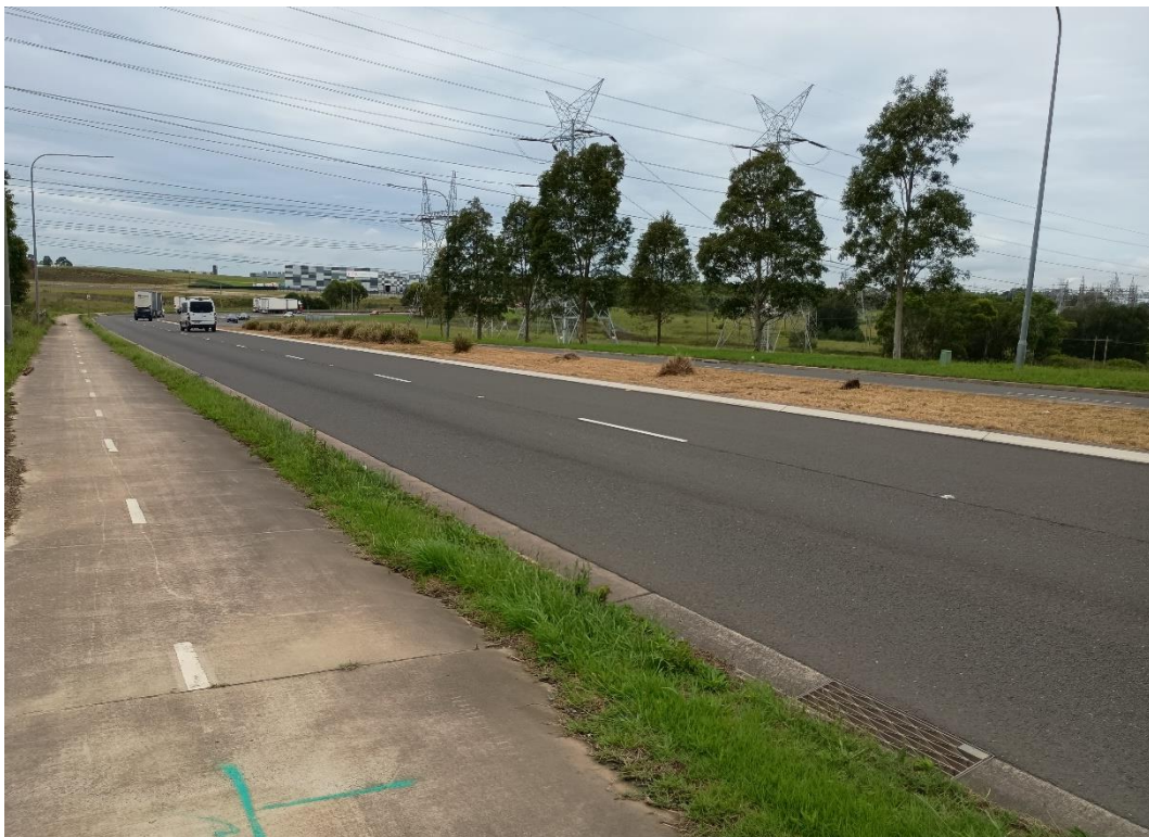
Photograph 10: Lenore Road at Service Alignment Chainage CH 1500 m Facing East
