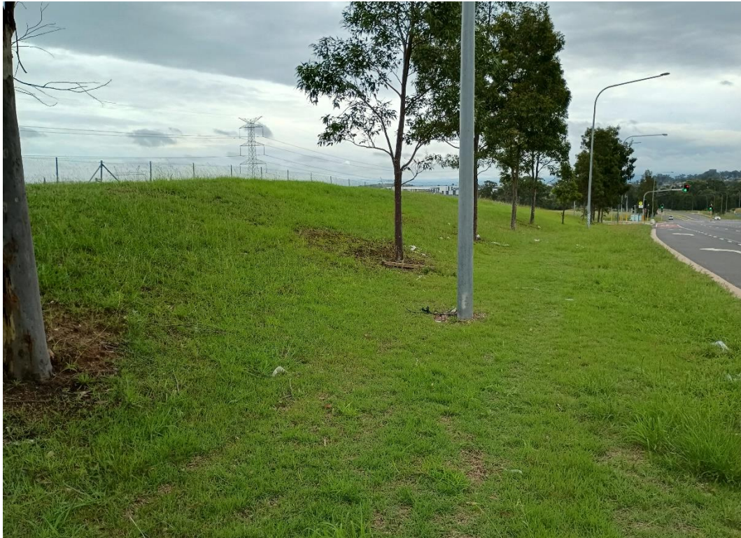
Photograph 5: Mounding Along Side of Road Between Service Alignment Chainage 900 m and 1060 m
