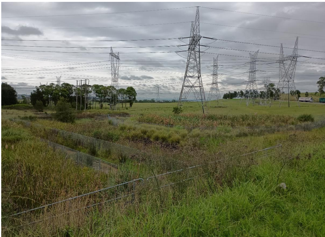
Photograph 6: Wetland at Between Service Alignment Chainage 90 m and 360 m
