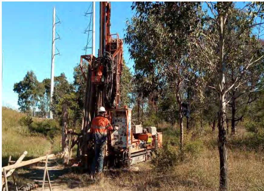
Photo 6 - Drilling rig at BH03 Location
