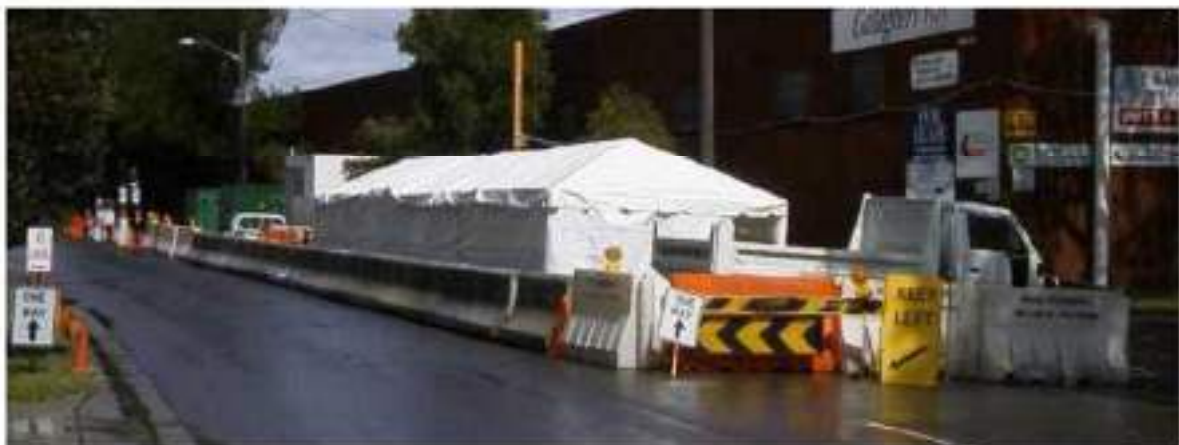
Figure 5; Example of cable pulling and cable joint works
