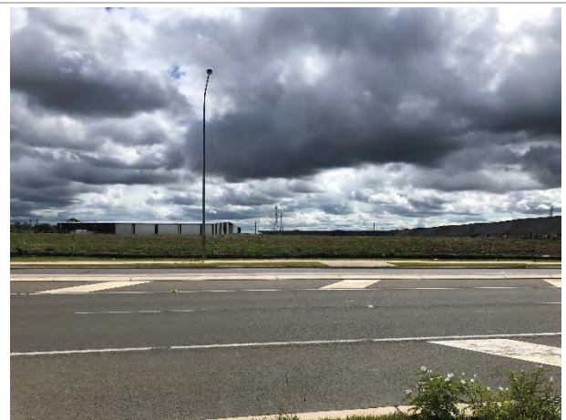
Chainage 14.1-45.2 (Lenore Drive crossing)
