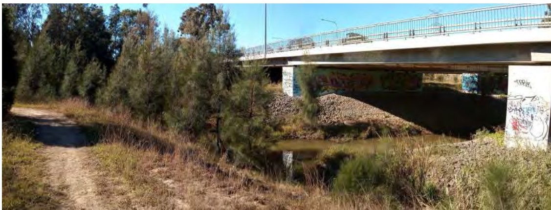
Photo 3 - General Site Conditions - View of the creek and bridge near BH03
