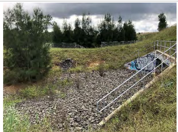
Culvert drainage in between Ropes Creek and basin
