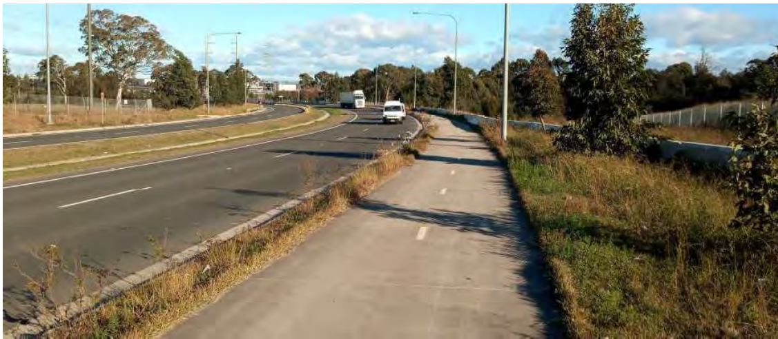
Photo 1 - General Site Conditions - Lenore Drive Near BH05
