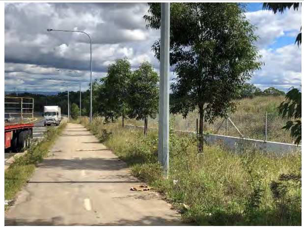
Shared pathway (viewed from near Chainage 1226.7)
