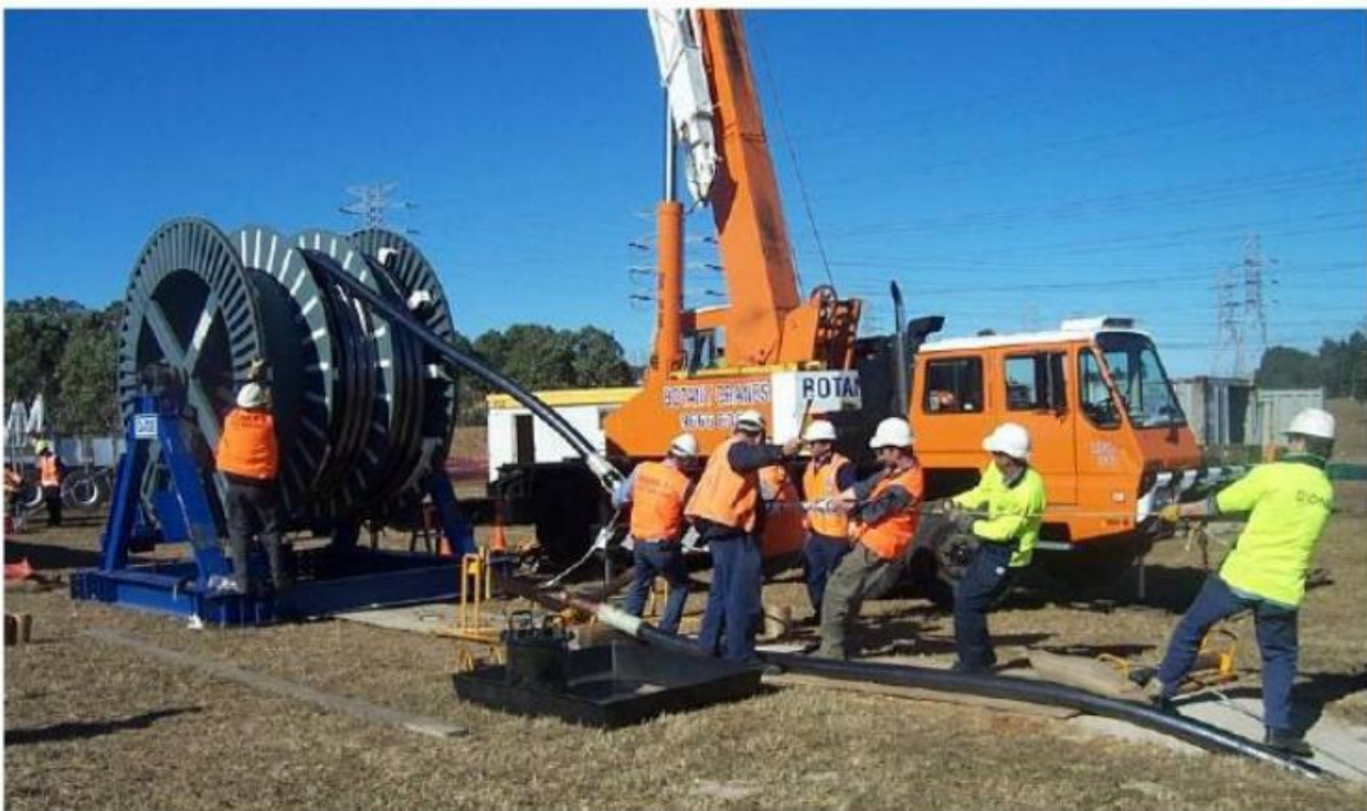
Figure 12 Example of Cable Pulling and Cable Joint Works
