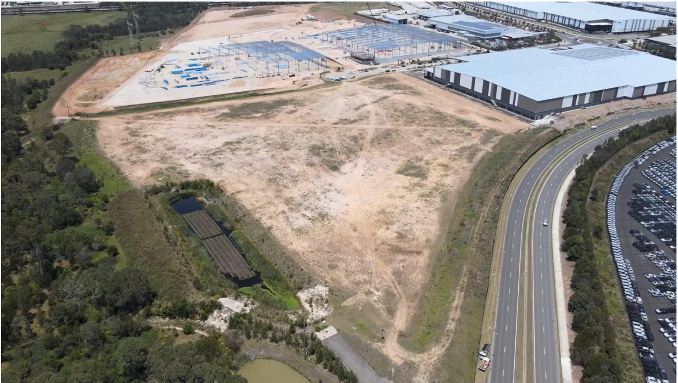
Picture 1 Aerial view of site, facing south-west
