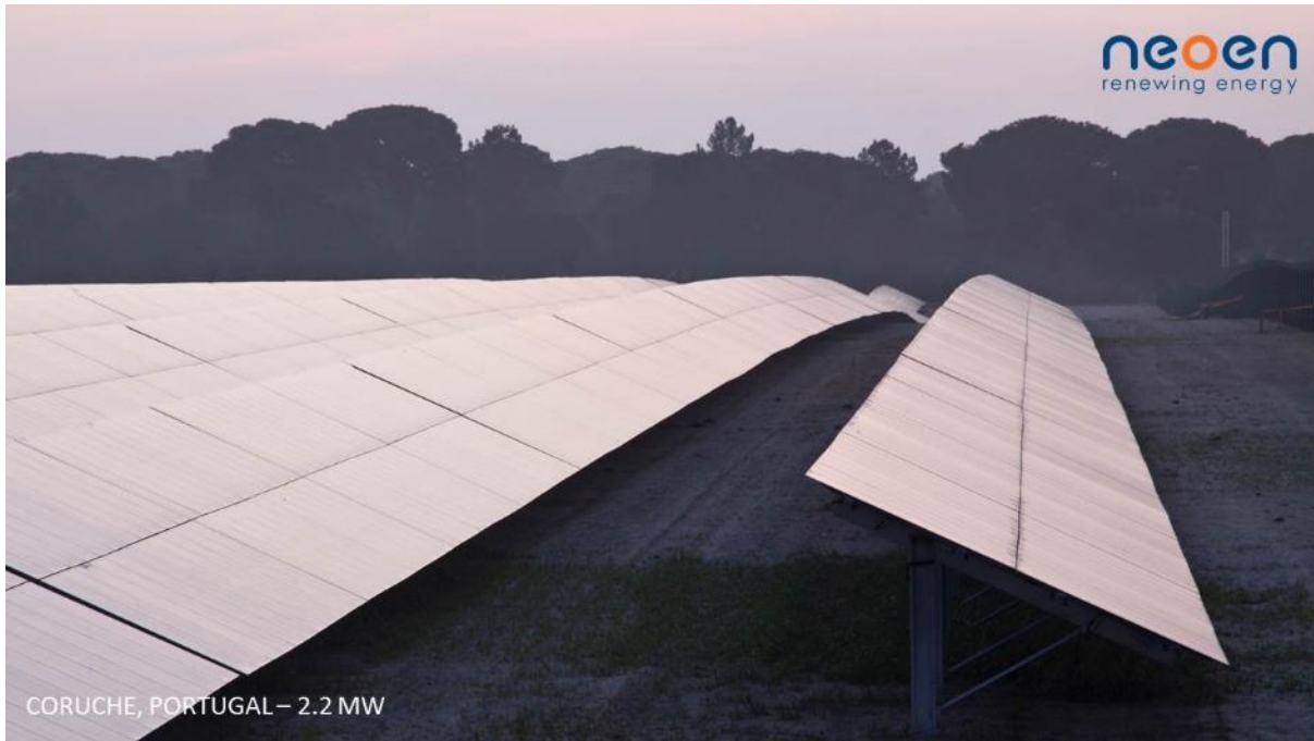
Figure 2-2 Example of south-facing fixed-tilt mounting system with thin-film technology in Europe (installation in Australia would face the north)
