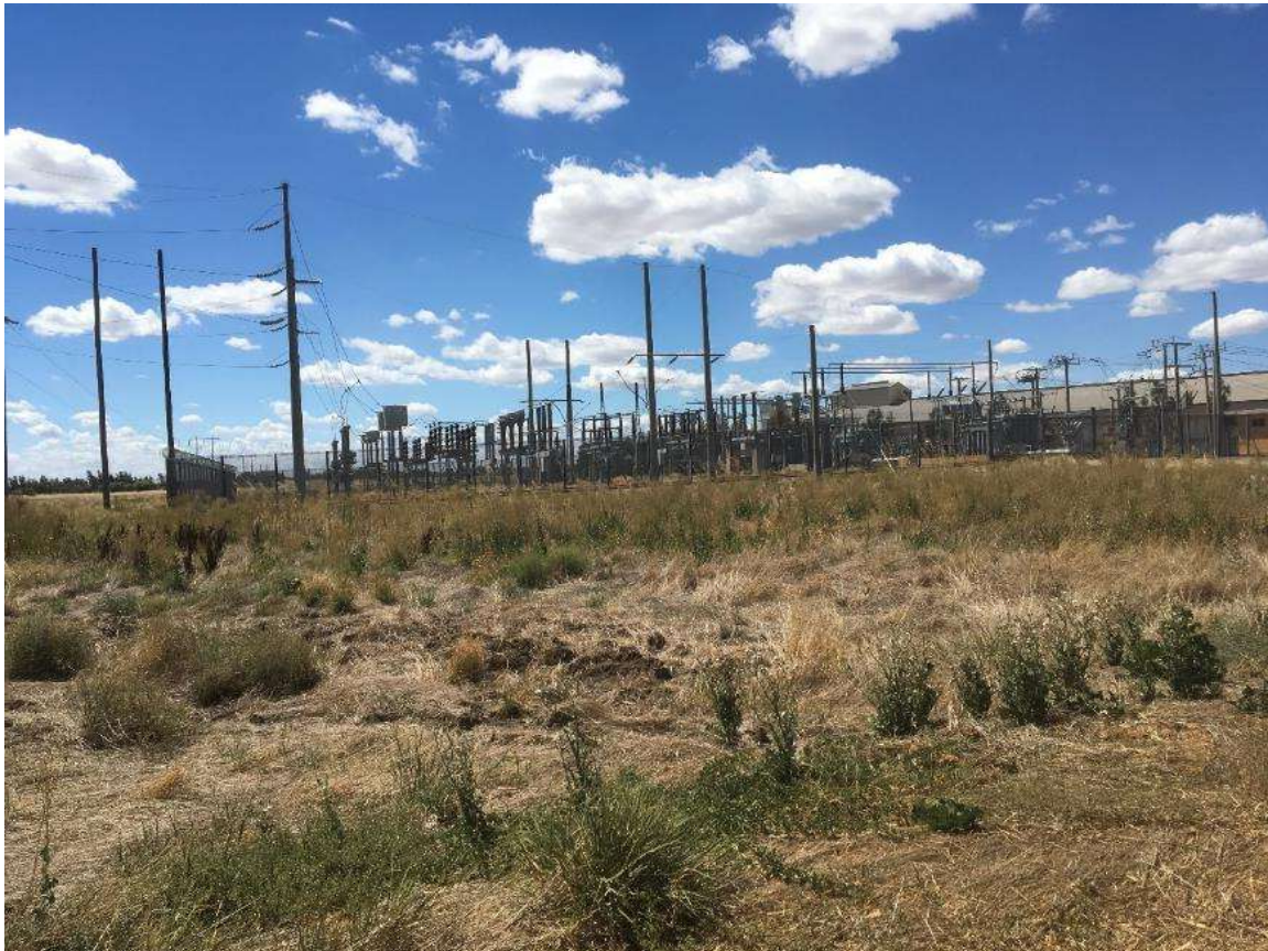
Figure 3-5 Existing substation accessed from Ercildoune Road.
