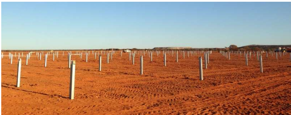
Figure 3-1 Example of poles driven into the ground on a Neoen solar project in Western Australia
