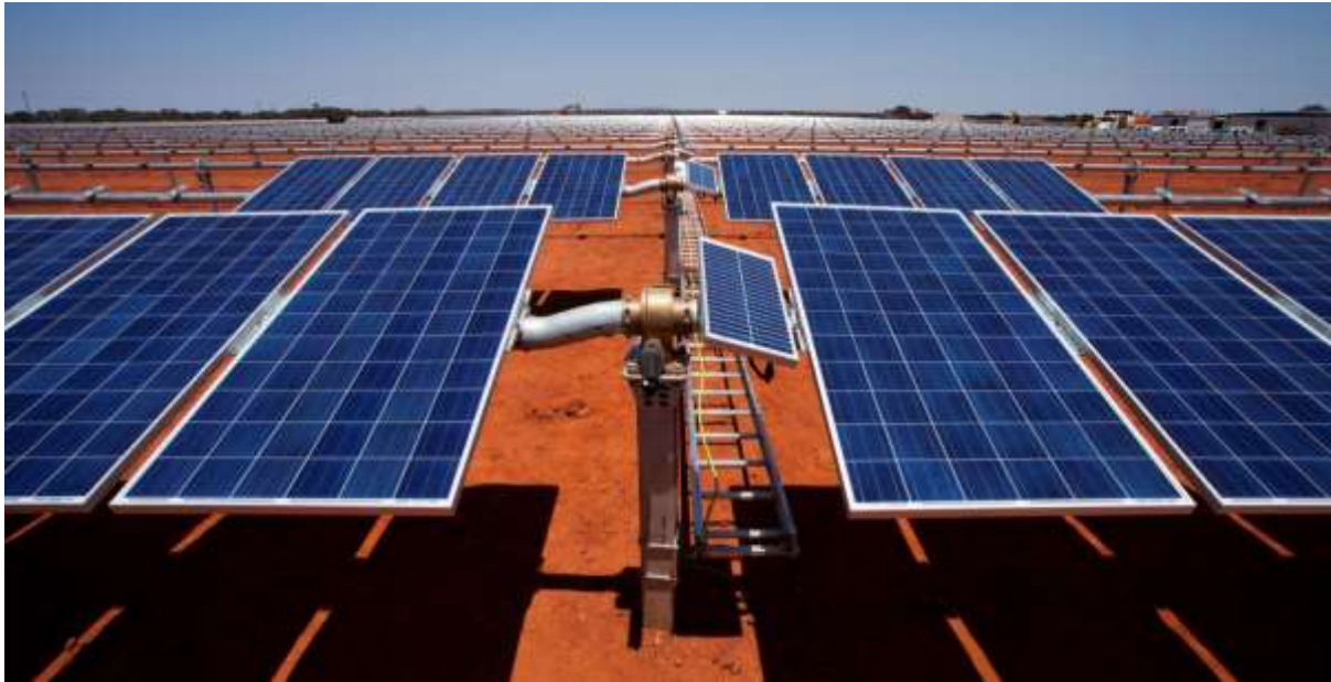
Figure 3-3 Example of a single-axis mounting system after panel installation.
