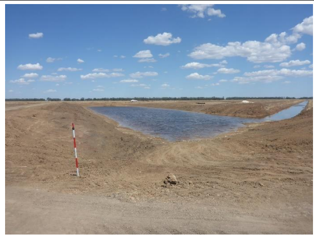
Plate 2 View south-west of the irrigation channels in the project area.
