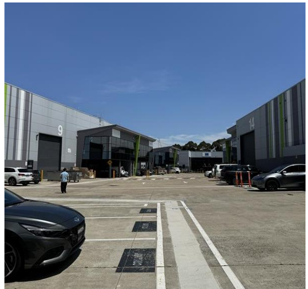
Picture 4 View of the eastern half of the site from the car park
