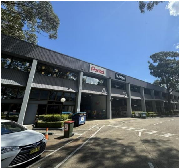
Picture 3 Rear building on the site viewed from the north
