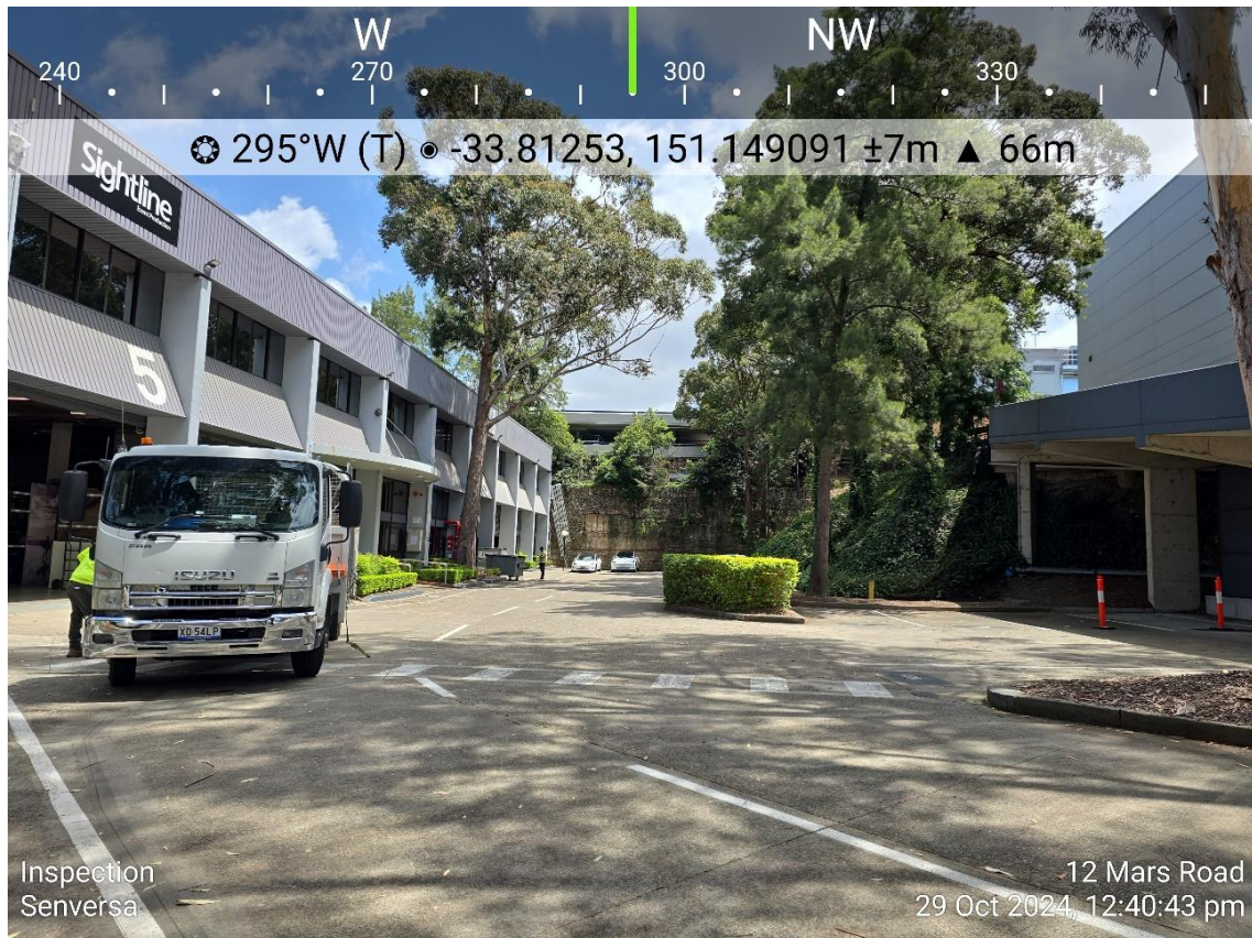
Photo 5. Driveway Throughout Estate
