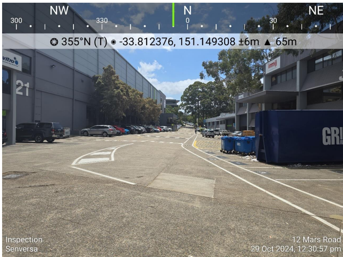
Photo 6. Driveway Throughout Estate
