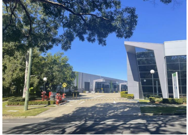
Picture 2 The site, access way to units 8-19
