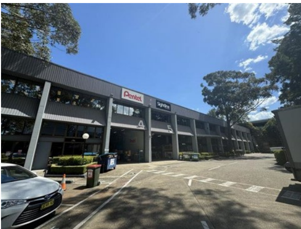
Picture 3 Rear Building on the site viewed from the north
