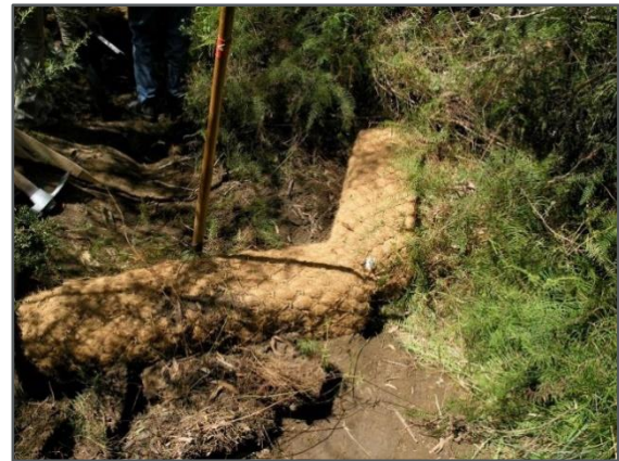
Plate 7-5 - Square Coir Logs for Knickpoint Control
