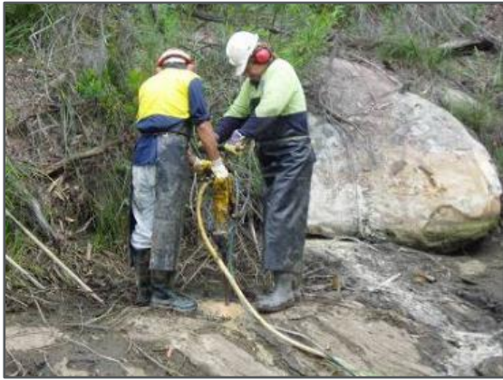
Plate 7-3 - Drilling into Bedrock to Form Grouting Holes
