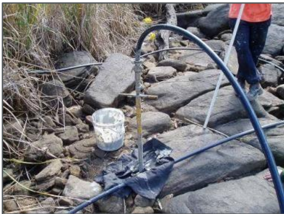
Plate 7-4 - Example of Rockbar Grouting Injection Undertaken in the Georges River
