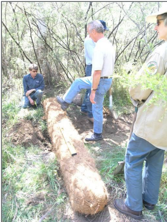
Plate 7-7 - Round Coir Logs Installed to Spread Water Source: Good et al. (2010).
