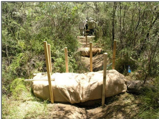
Plate 7-6 - Coir Log Dams Constructed at Intervals with Wrapping of Fibre Matting Source: Good et al. (2010).
