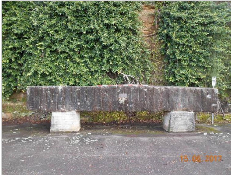
Plate 16: An example block of cyclopean masonry next to Cordeaux Dam wall (Niche 2017)
