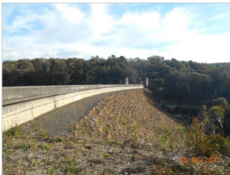
Plate 23: The downstream face of Avon Dam wall with its 1970s modifications (Niche 2017)
