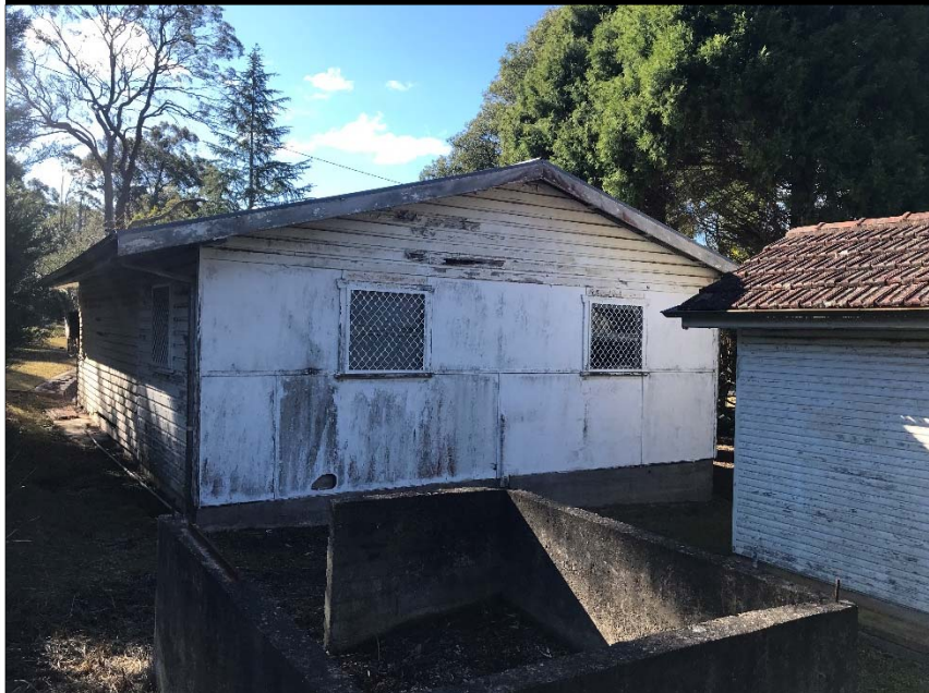
PHOTOGRAPH D: AREA 6, POTENTIAL ASBESTOS CEMENT CLADDING
