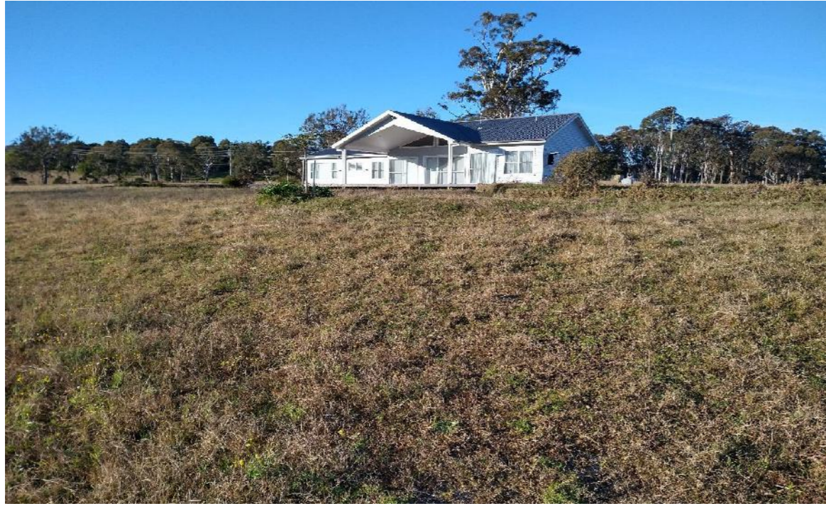
Photo 1: General view of the residential dwelling northern facade, looking east.
