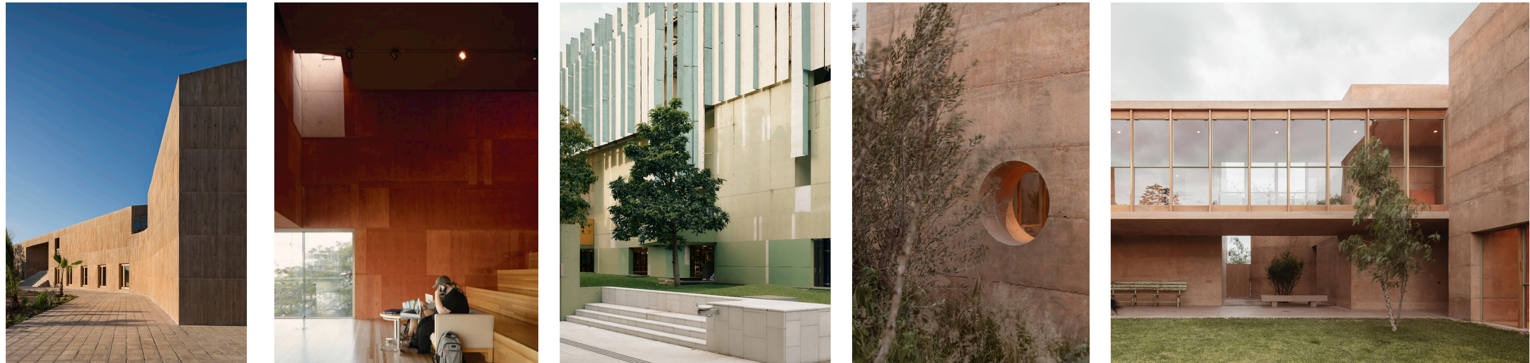
Grounding pigmented concrete panels to lower level in natural earthy colours to add warmth. Variation in colour/texture to add interest and human scale.
