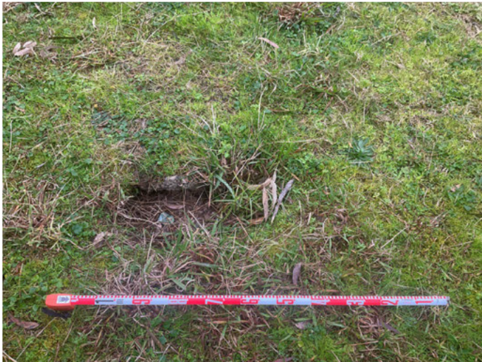
Figure 5-8: Partially embedded concrete fragment south of the data centre building. Located within SU-01, facing east.
