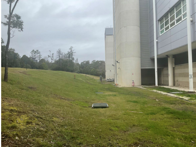
Figure 5-4: View across the slope and terracing to the north of the data centre building. Located within SU-01, facing east.
