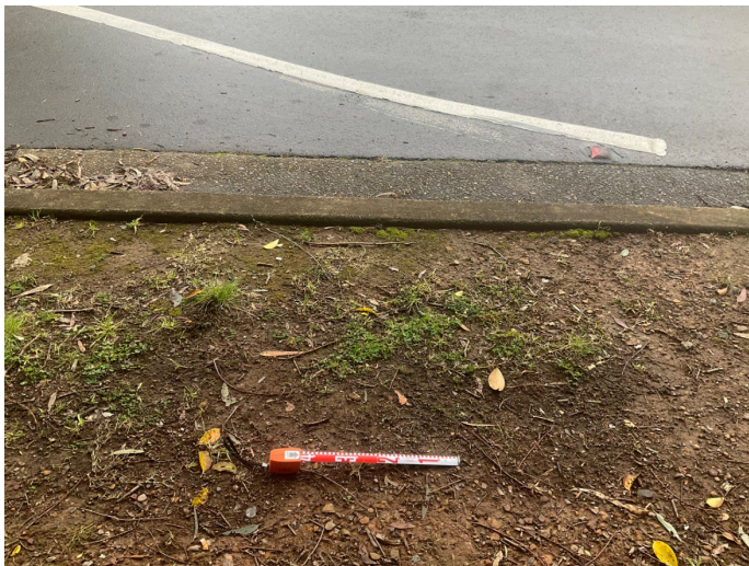
Figure 5-14: Ground surface and fragments of stone, brick and concrete within area of exposure along edge of Brookhollow Avenue. Located to the east of SU-02, facing east.
