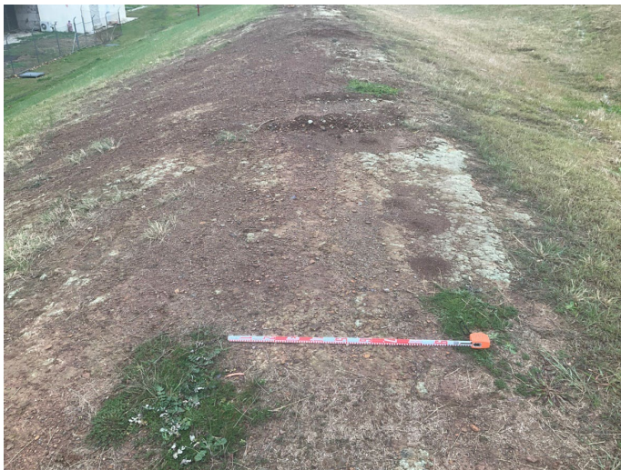
Figure 5-11: Area of exposure at top of terrace. Located in SU-02, facing west.
