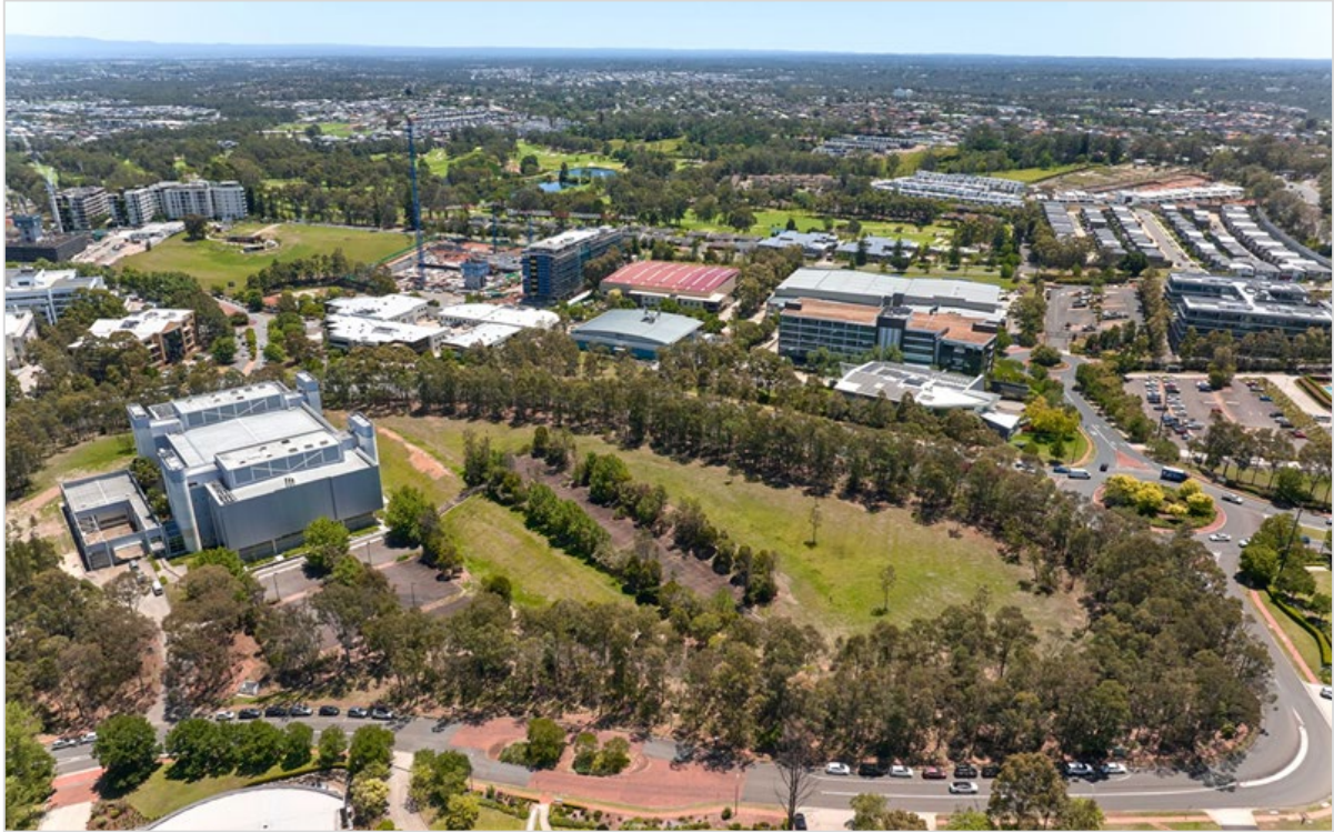
Figure 3-7: Aerial photograph of the 3 Brookhollow Avenue site. (Source: DataCentreDynamics. 2025)
