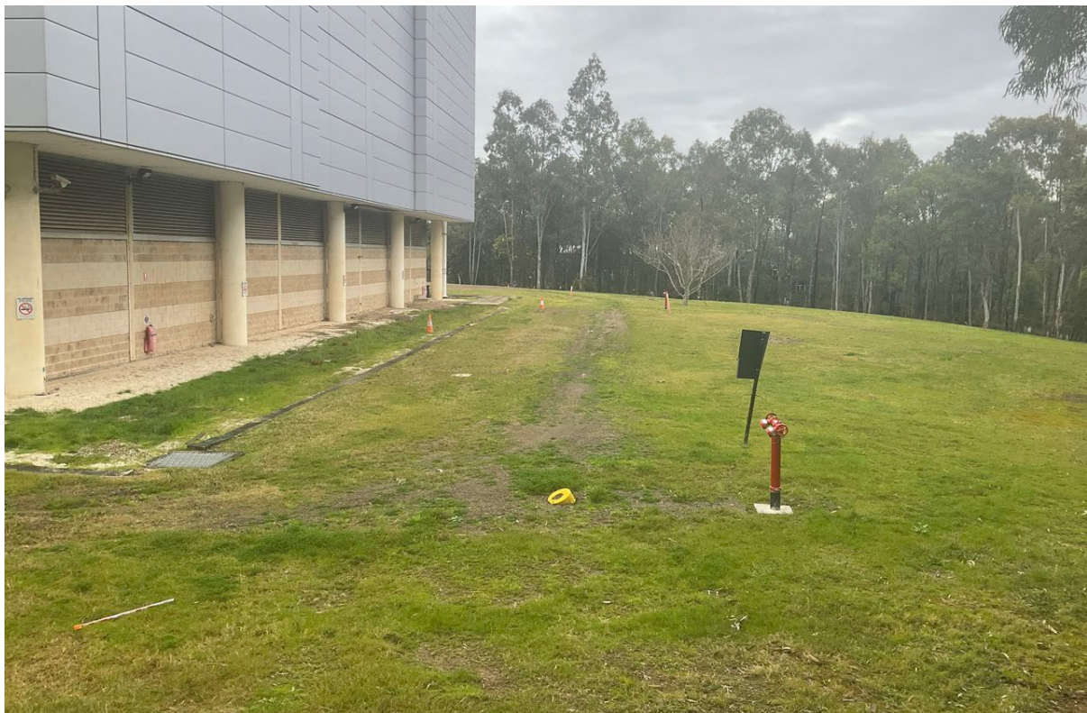
Figure 3-11: View across the northern side of the data centre of 3 Brookhollow Avenue site, facing east (Source: Everick Heritage. 2025).
