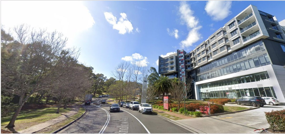
Figure 3-5: View along Brookhollow Avenue, facing east. (Source: Google. 2024)
