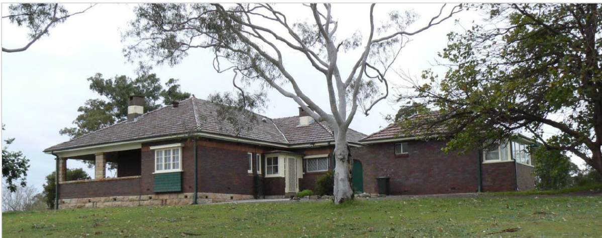
Figure 3-14: View of St Joseph's Novitiate, facing southeast. (Source: The Hills Shire Council. 2007)
