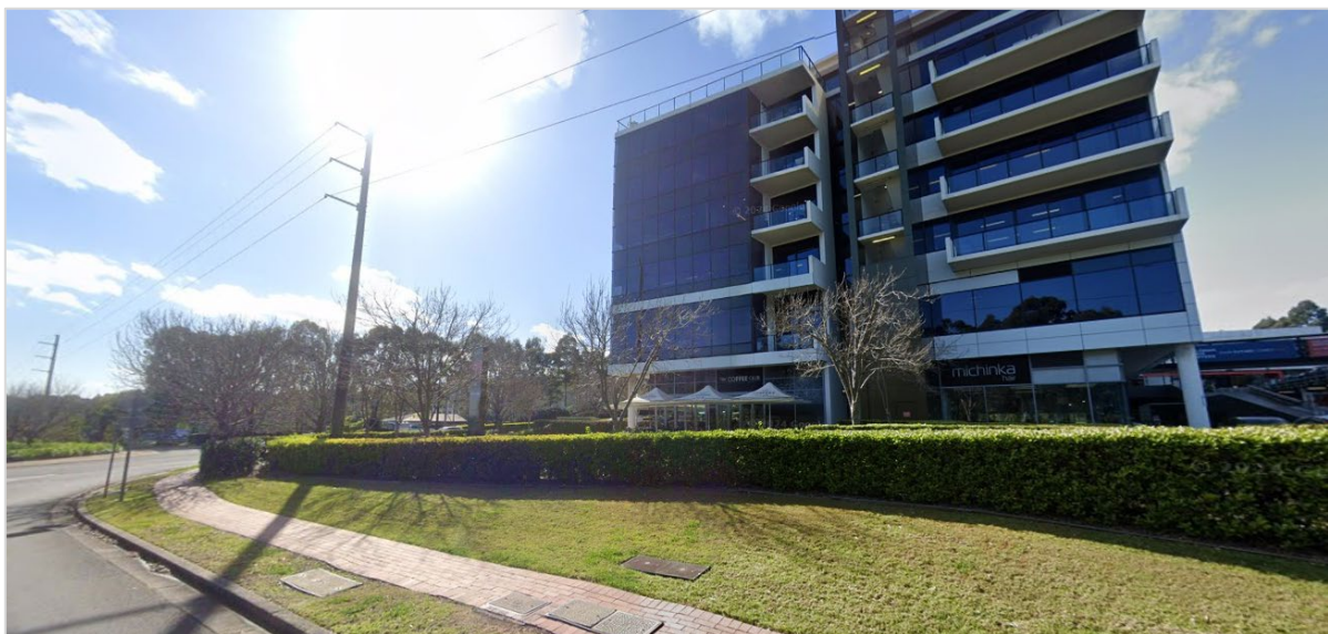
Figure 3-6: View across Windsor Road, facing northeast. (Source: Google. 2024)
