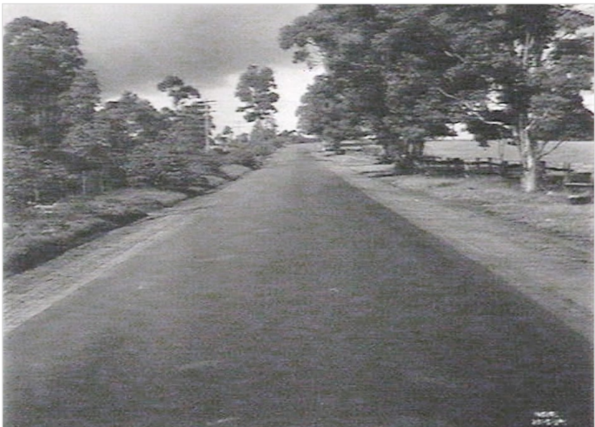
Figure 2-8: Photograph of the Baulkham Hills to Box Hill section of Windsor Road, taken in 1930. (Source: State Library of NSW. Call Number: Government Printing Office 1 - 01877, Original negative held by State Archives & Records Authority of New South Wales.)
