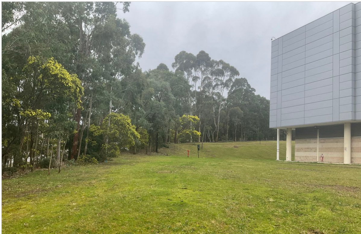
Figure 3-9: View along the western side of the data centre building, facing north. (Source: Everick Heritage. 2025)
