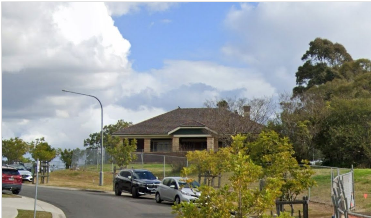
Figure 3-12: View of St Joseph's Novitiate, facing northwest. (Source: Google. 2024)
