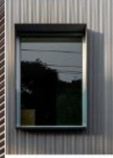
M01 - METAL CLAD WINDOW SHROUD
