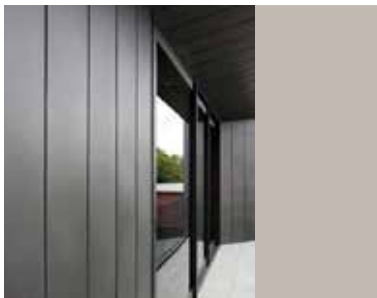
Metal cladding external wall with interlocking seam in Nickel Pearl Matt.
