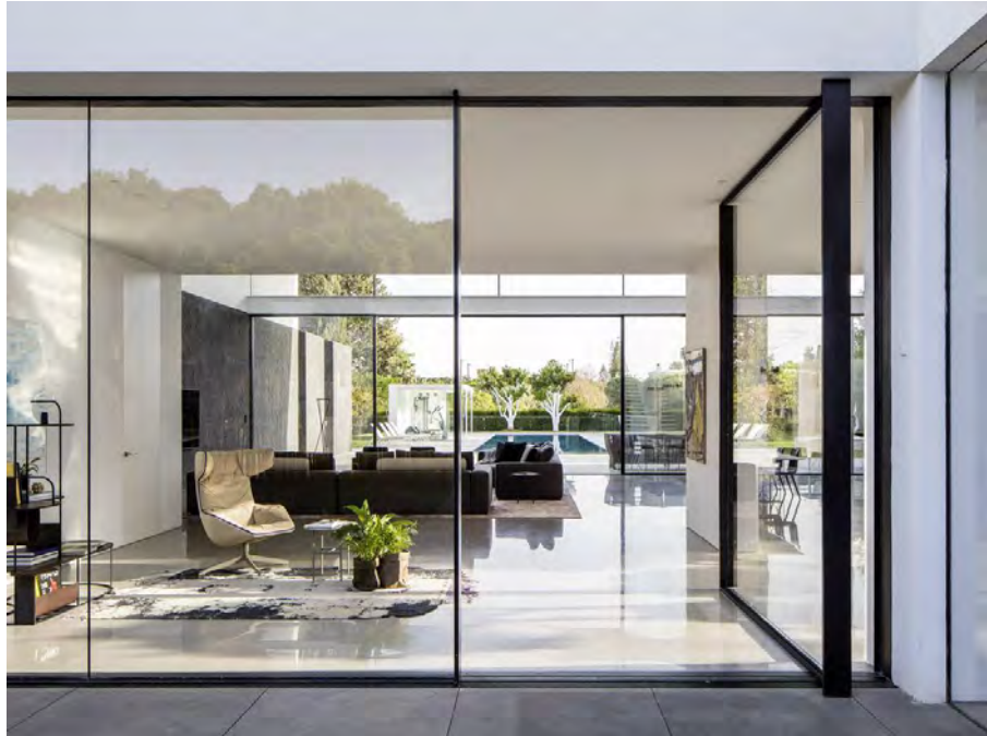
AFG ALUMINIUM FRAMED GLAZING POWDERCOAT- MONUMENT MATT OR SIMILAR
