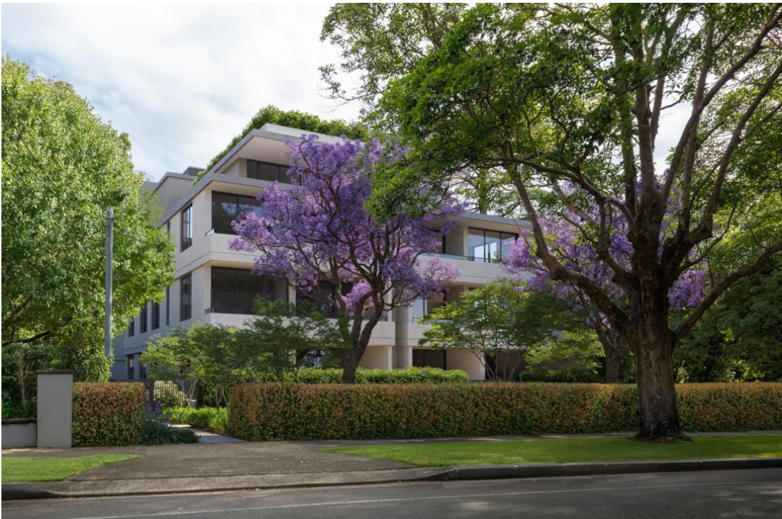
Figure 5: Proposed built form outcome once completed (Source: PBD Architects)
