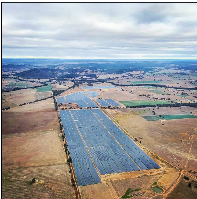
Figure 2-1 Beryl Solar Farm post construction (courtesy of Tranex Solar)
