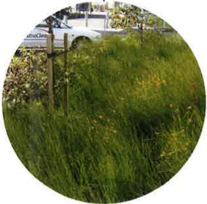
Planted swales in centre median to cleanse stormwater runoff from carpark
