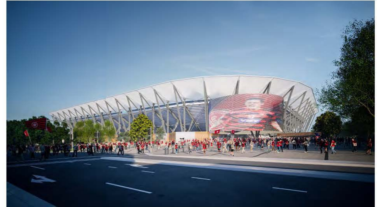
6.9.2 Expressive urban character of entrances: eastern facade
