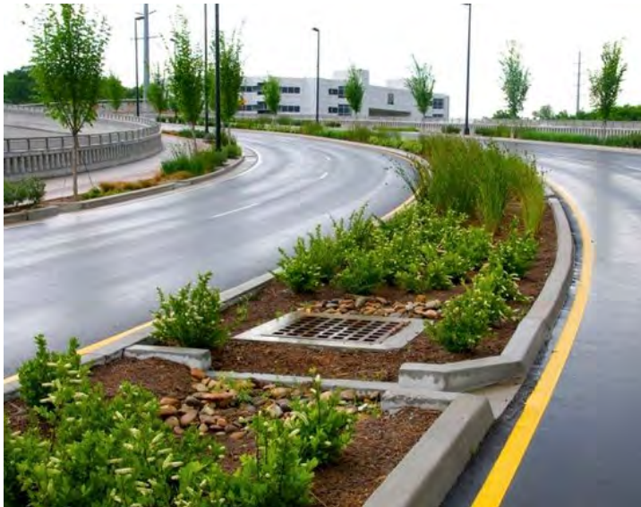
Figure 10 - Integrated Car Park Bio-Swale
