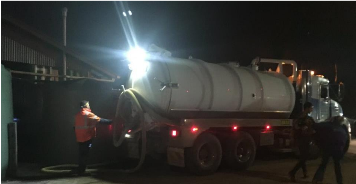
Photograph 5: Vacuum extraction of wastewater from temporary poly storage tanks at an amenities block.
