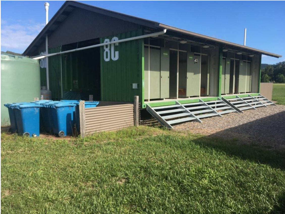
Photograph 1: Amenities 8, consisting of shower cubicles on RH side and compost toilets on LH (far side of amenities). Green poly tanks on LH side are rainwater collection tanks.
