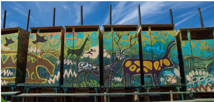
Photograph 12: Boom Festival compost toilets.
