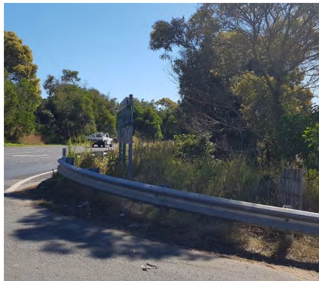
Photo 4.2 Gate D looking north along Tweed Valley Way
