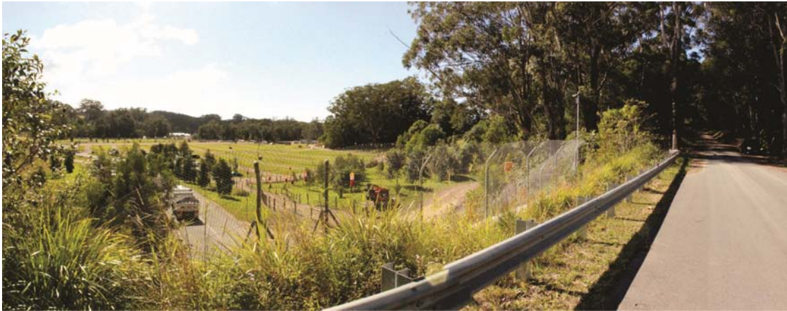
Above: View from the overpass on Jones Road towards the transport hub
