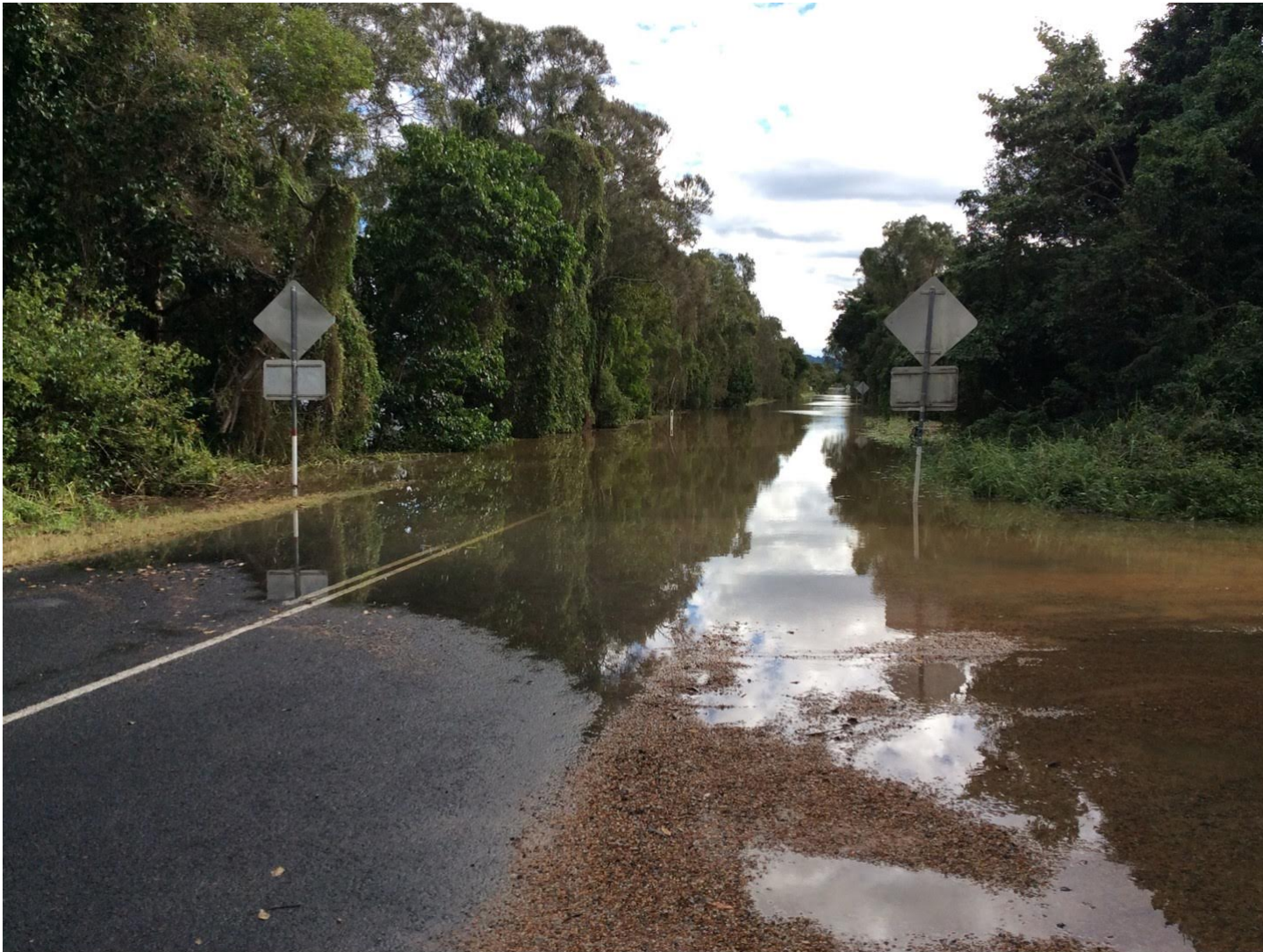
5 th June, 2016 taken on Wooyung Road next to caravan park, looking west on same day.
