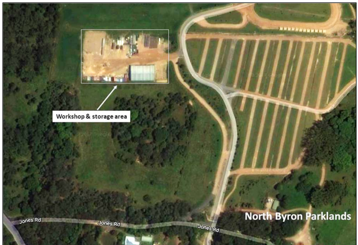
Figure 14 NBP Workshop & Storage
