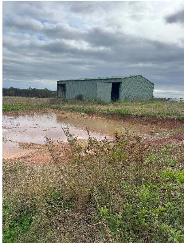
Figure 15 – View of the extant corrugated steel shed at 165 Lawson Road from the former location of the Federation era house, view north-west.
