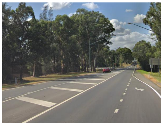
Figure 2-8 Mamre Road, facing south (Source: Google Earth)
