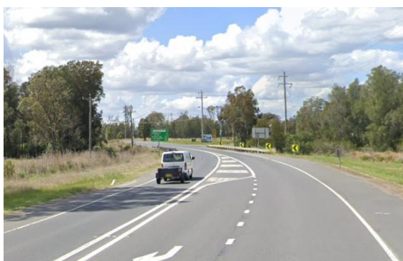
Figure 2-9 Elizabeth Drive, facing east (Source: Google Earth)
