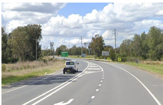
Figure 2-10 Elizabeth Drive, facing east (Source: Google Earth)
