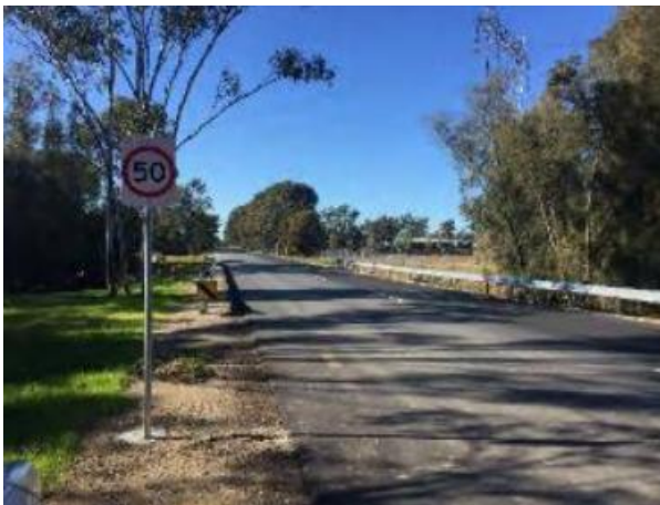
Figure 2-6 Patons Lane, facing west
