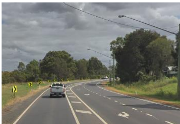
Figure 2-8 Mamre Road, facing north (Source: Google Earth)
