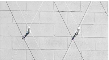
FACADE TRELIS Ronstan climbing frame to facade to support vertical planting
