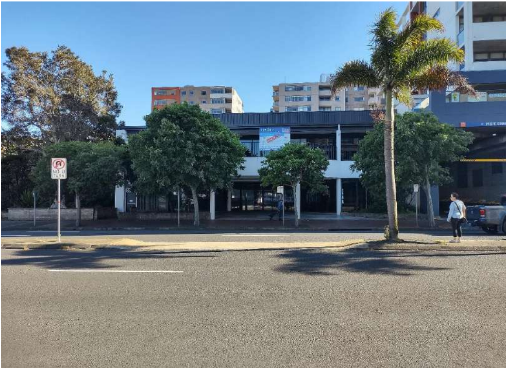
Photo 1: Site facade, viewed from the south
