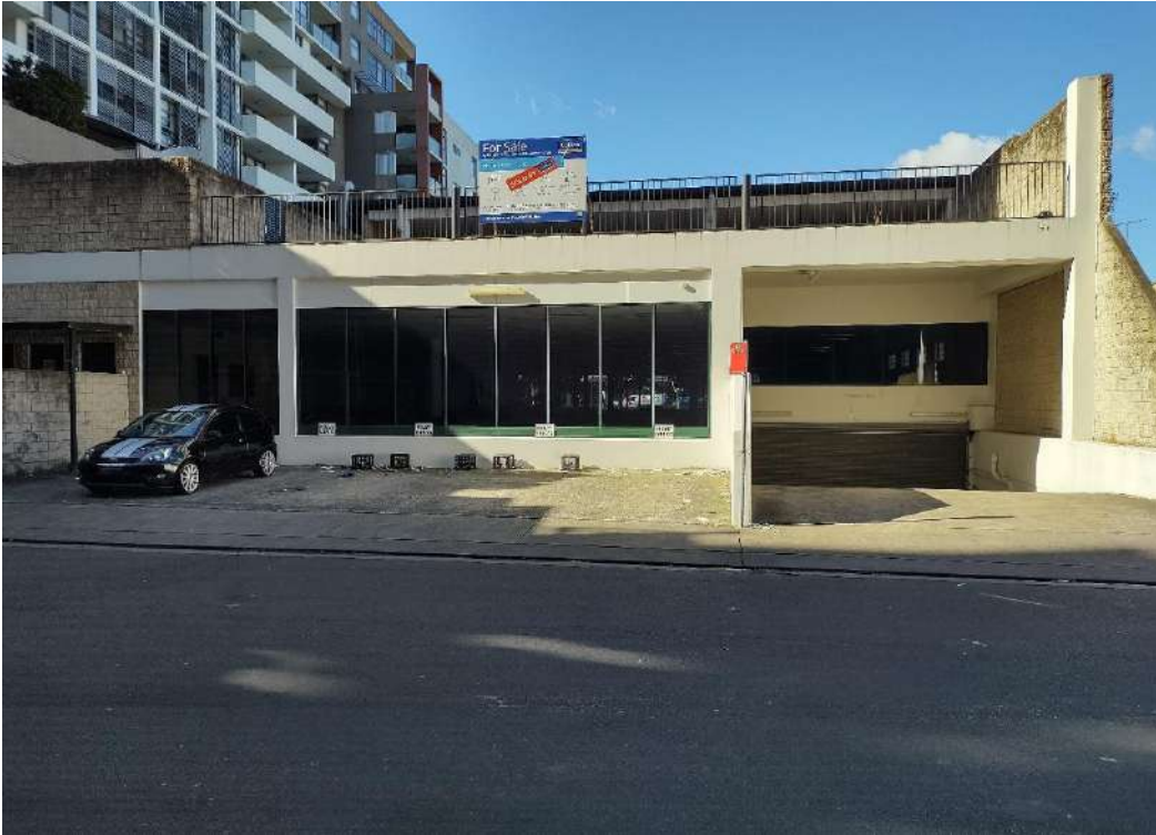
Photo 3: Rear entrance to building and basement, viewed from the north
