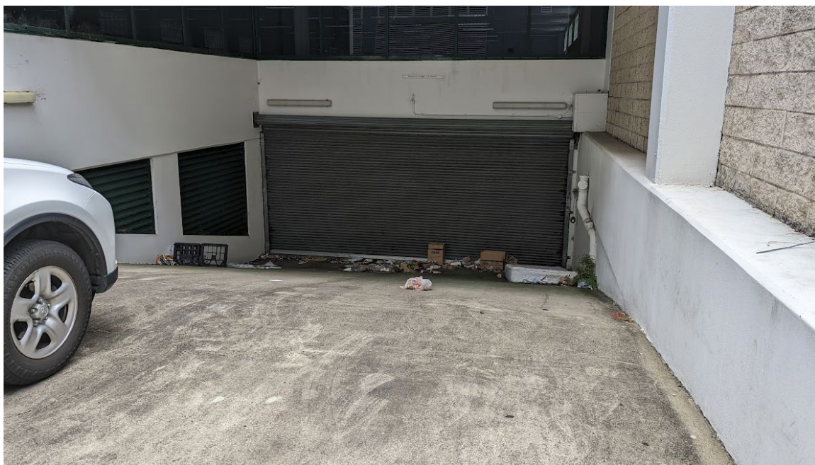
Figure 2 Existing vehicle access driveway
