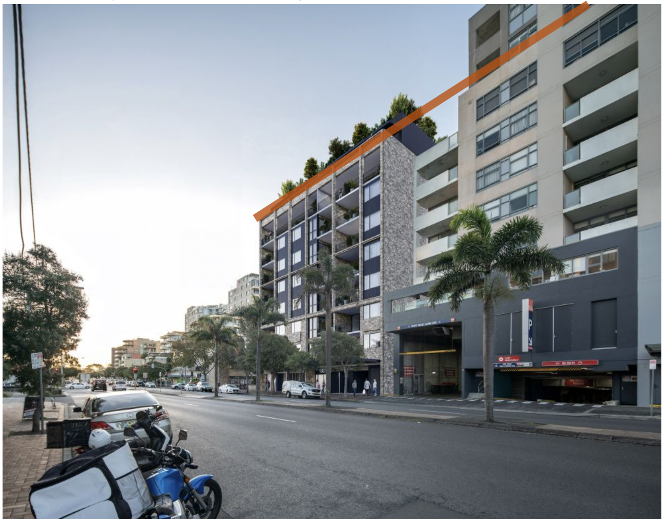
FIGURE 10: PHOTOMONTAGE OF MAROUBRA PARADE FRONTAGE LOOKING WEST (DJRD ARCHITECTS) WITH ORANGE LINES INDICATING THE DOMINANT STREET WALL HEIGHT
