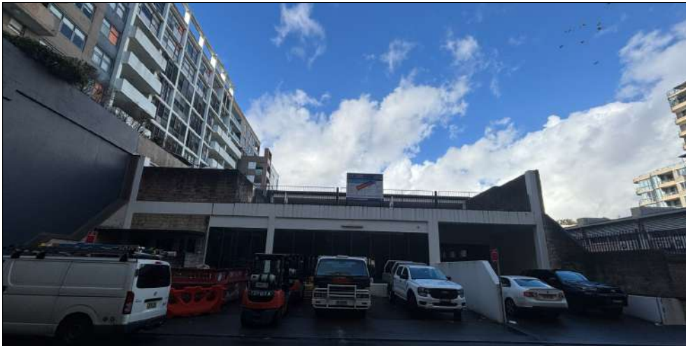
Figure 17: The rear elevation of the subject site from Piccadilly Place.
