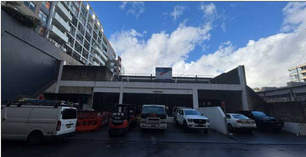
Figure 4: The rear elevation and balcony of the subject building from Piccadilly Place.
