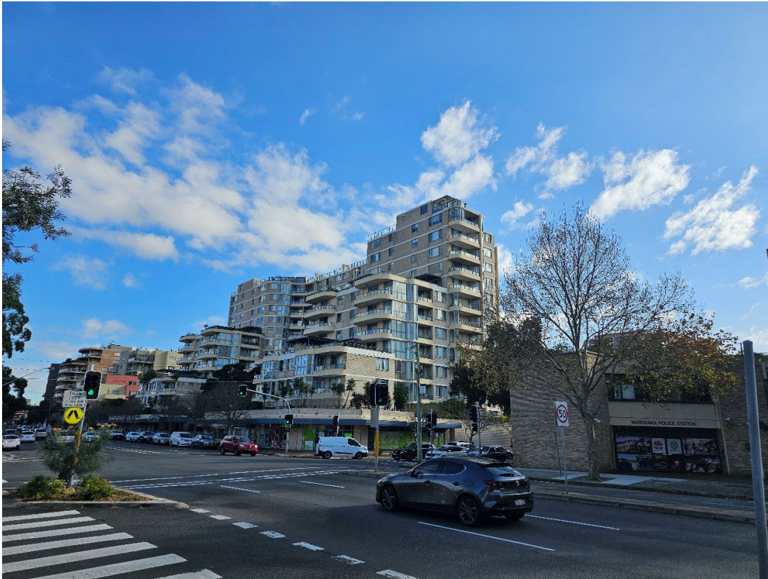
Figure 11: Maroubra town centre built form context west of the Site Source: Planning & Co
