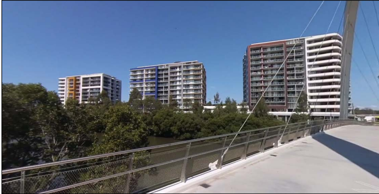
Figure 4. Existing shop top housing development up to 40m in height on the opposing side of Parramatta River (Source: PPUD)
