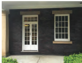
1 DETAIL Photo - Existing Elevation
