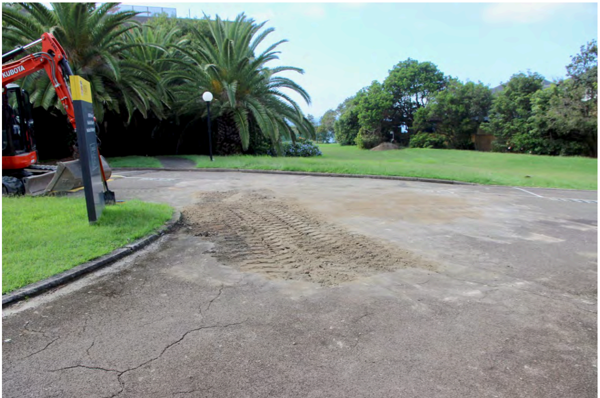
Figure 103: TT4 - After backfilling
