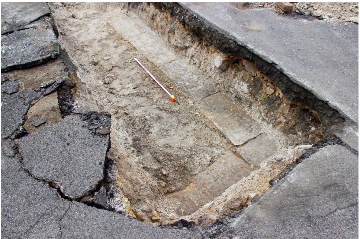
Figure 100: TT4 - In situ sandstone footings at base of trench
