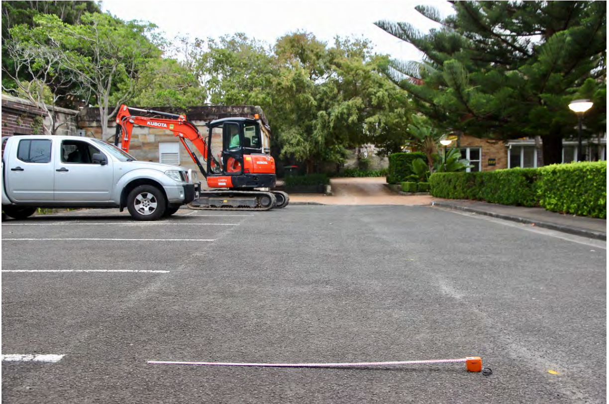
Figure 81: TT 2 - Prior to excavation
