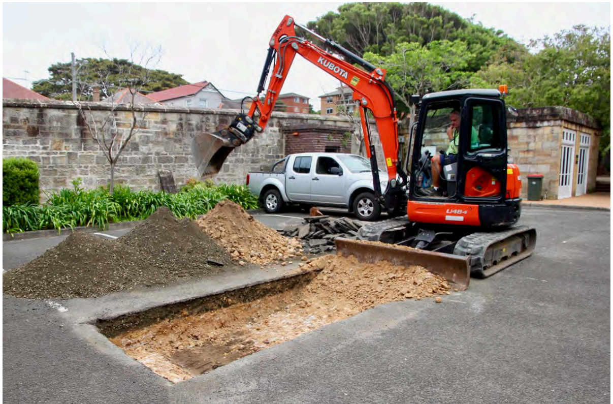
Figure 84: TT2 - Removal of compacted crushed sandstone fill
