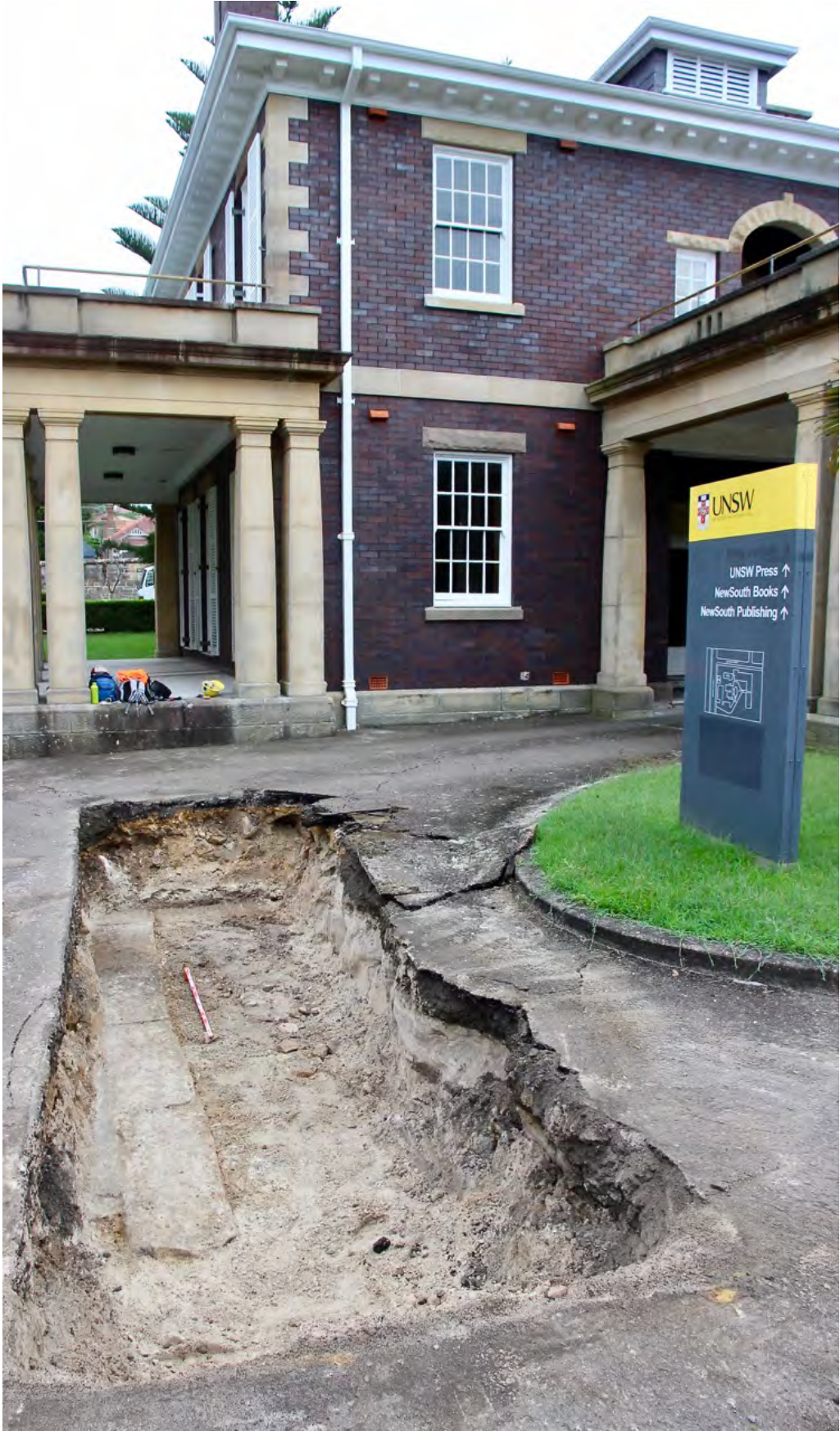
Figure 101: TT4 - In situ sandstone footings at base of trench
