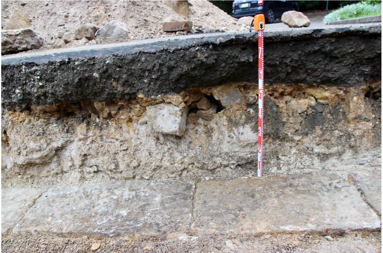
Figure 102: TT4 - Partial south section
