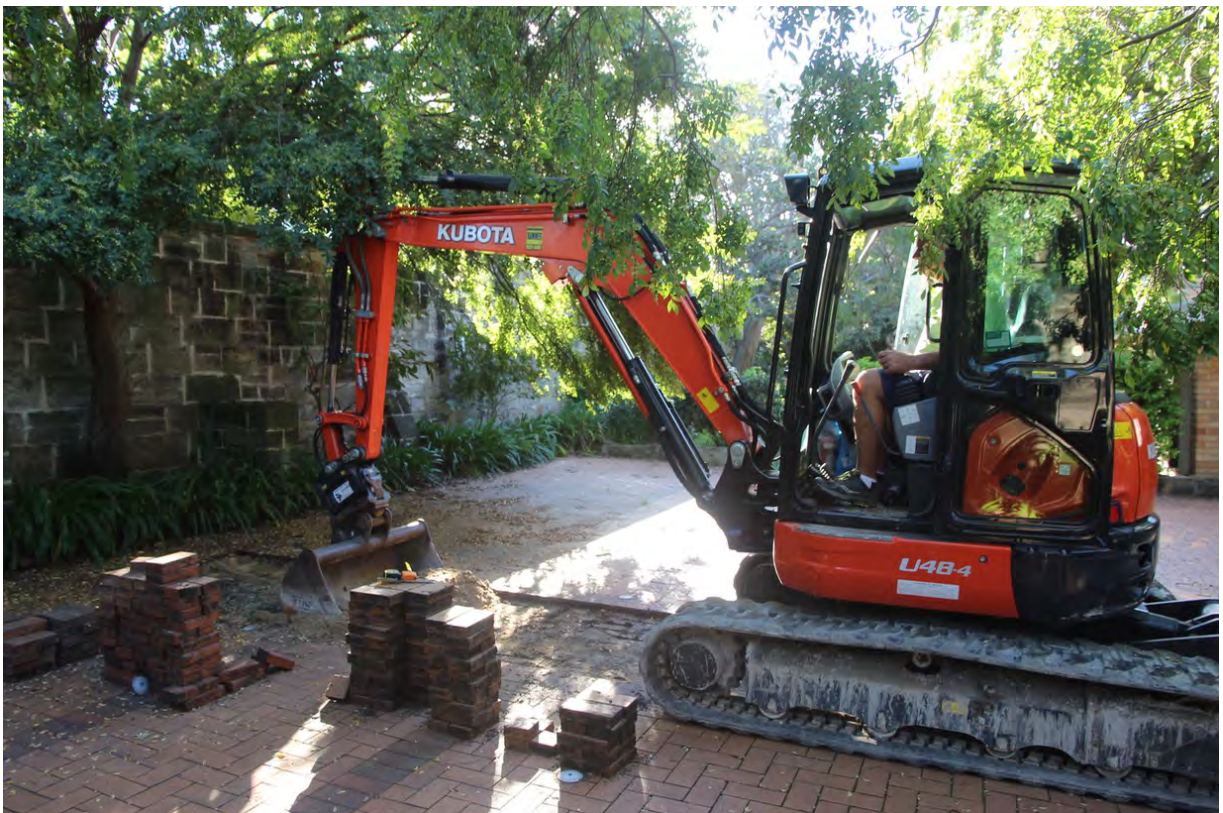
Figure 75: TT - Excavation in progress
