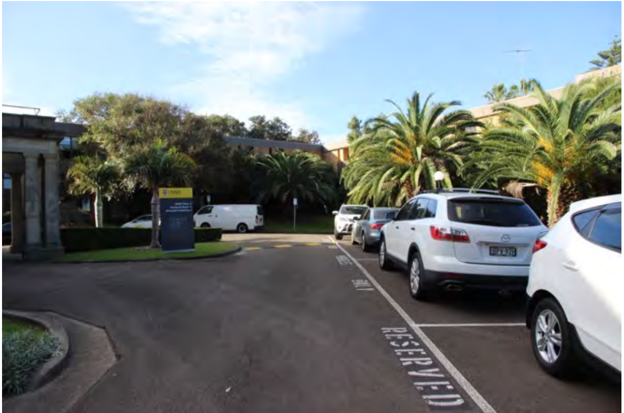
Figure 63: CliffBrook (portico at left with building CC4 at rear)
