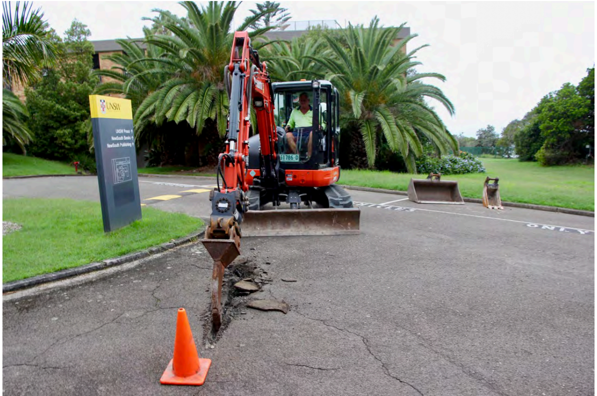
Figure 97: TT4 - Cutting surface bitumen
