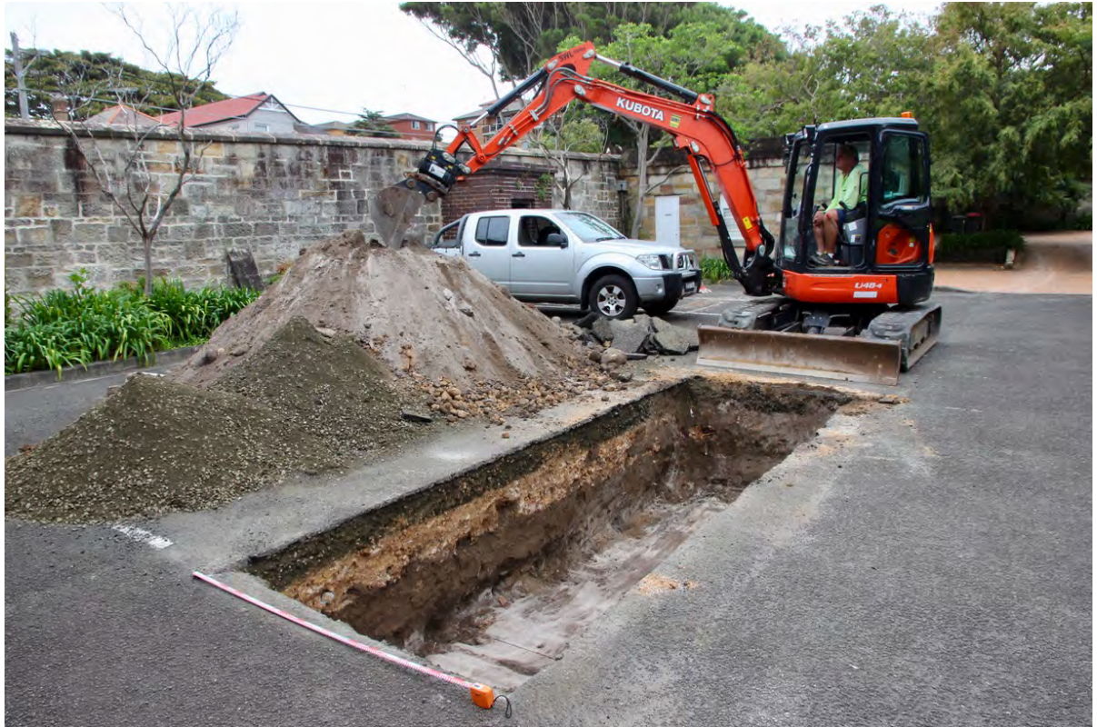
Figure 85: TT2 - Excavation at completion
