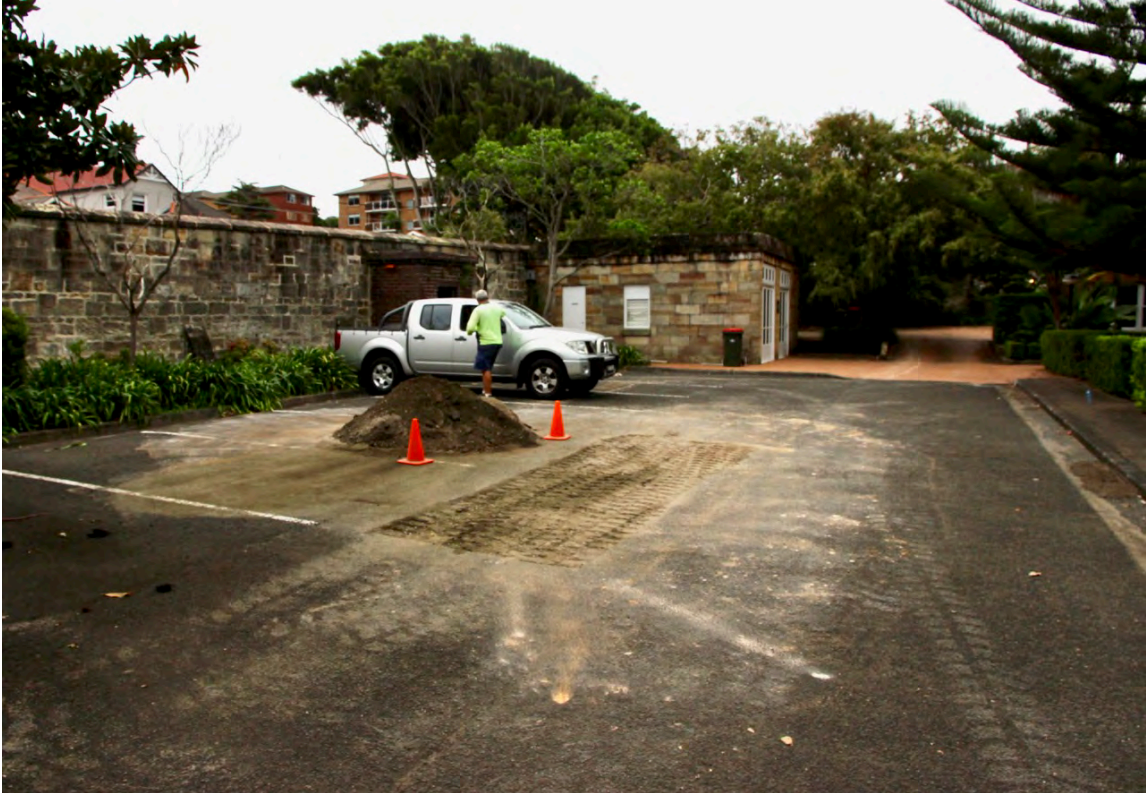
Figure 88: TT2 - After backfilling View SW - Dan Tuck 2017
