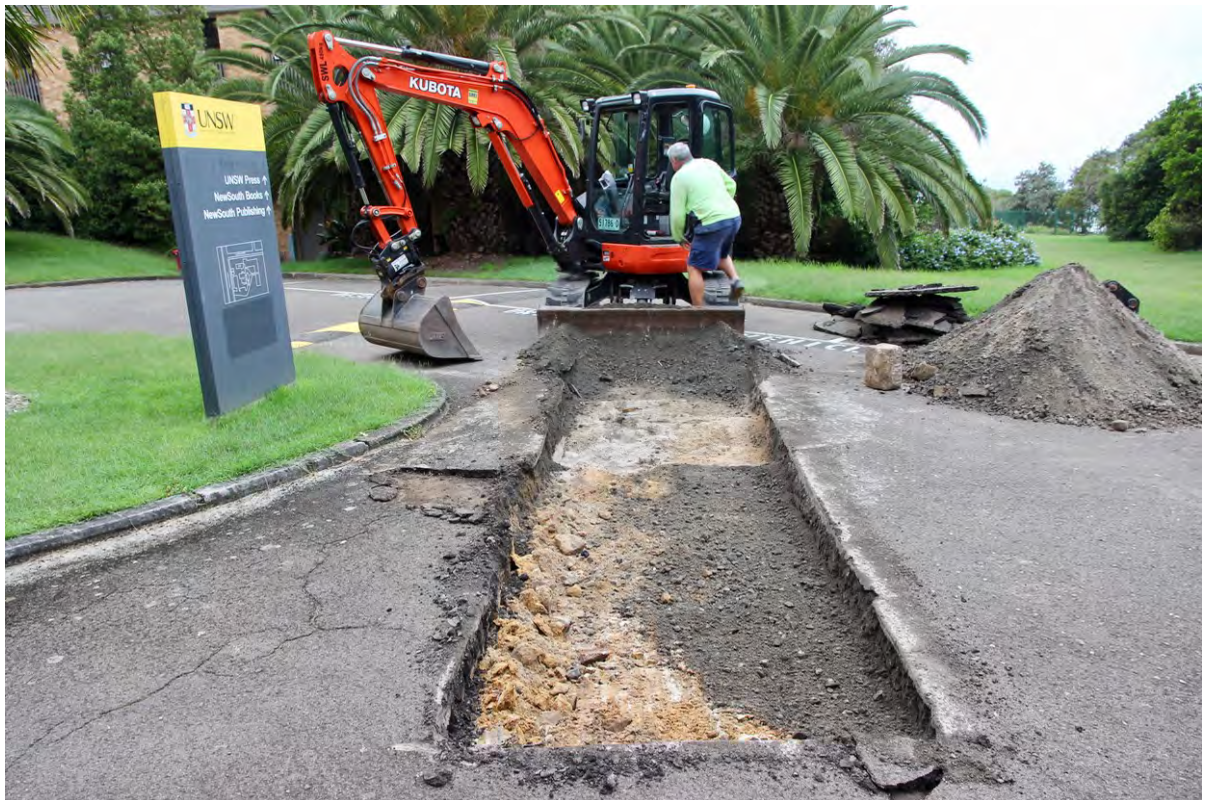
Figure 98: TT4 - Removal of bitumen & road base (with construction deposit exposed below)
