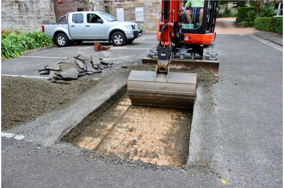
Figure 83: TT2 - Road base removal
