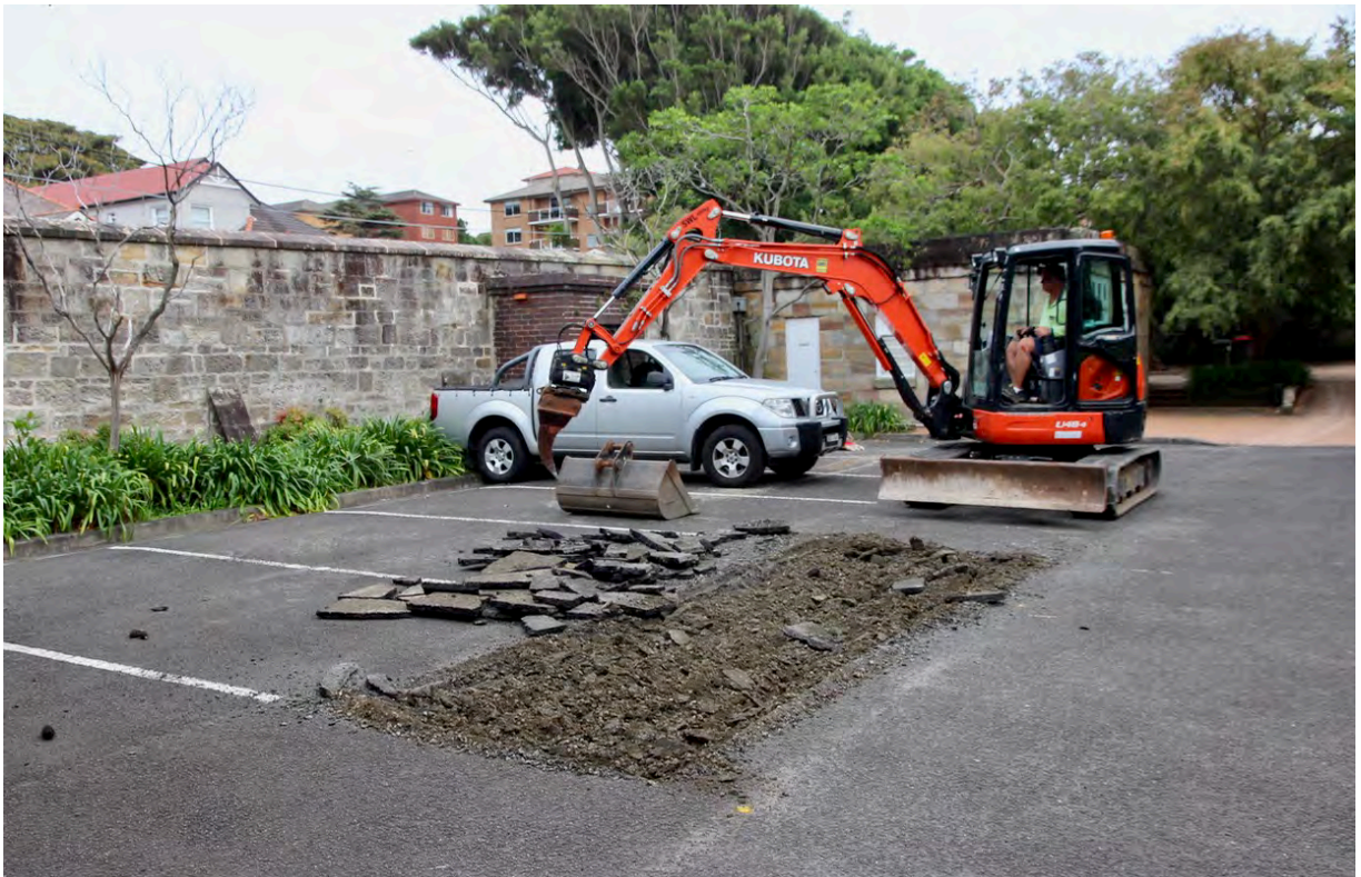
Figure 82: TT2 - Bitumen removal
