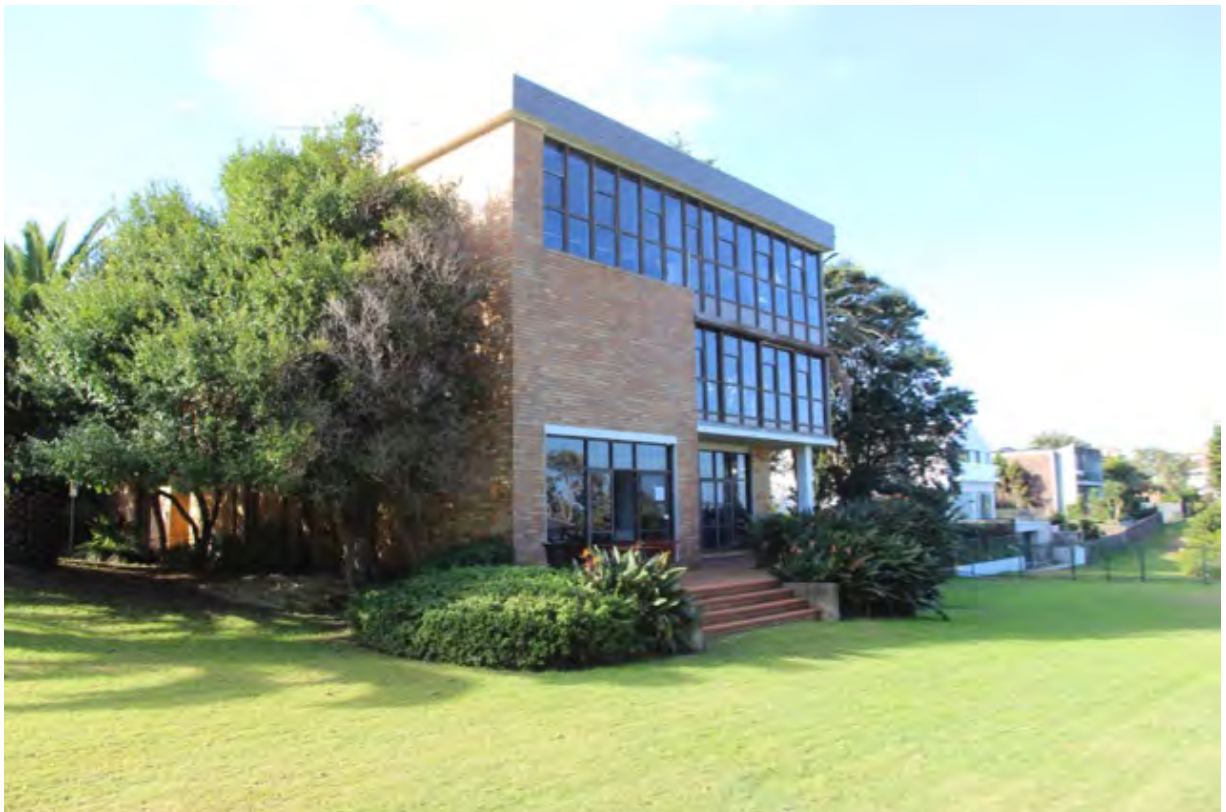
Figure 64: CliffBrook (building CC4 east wing & open lawn area)
