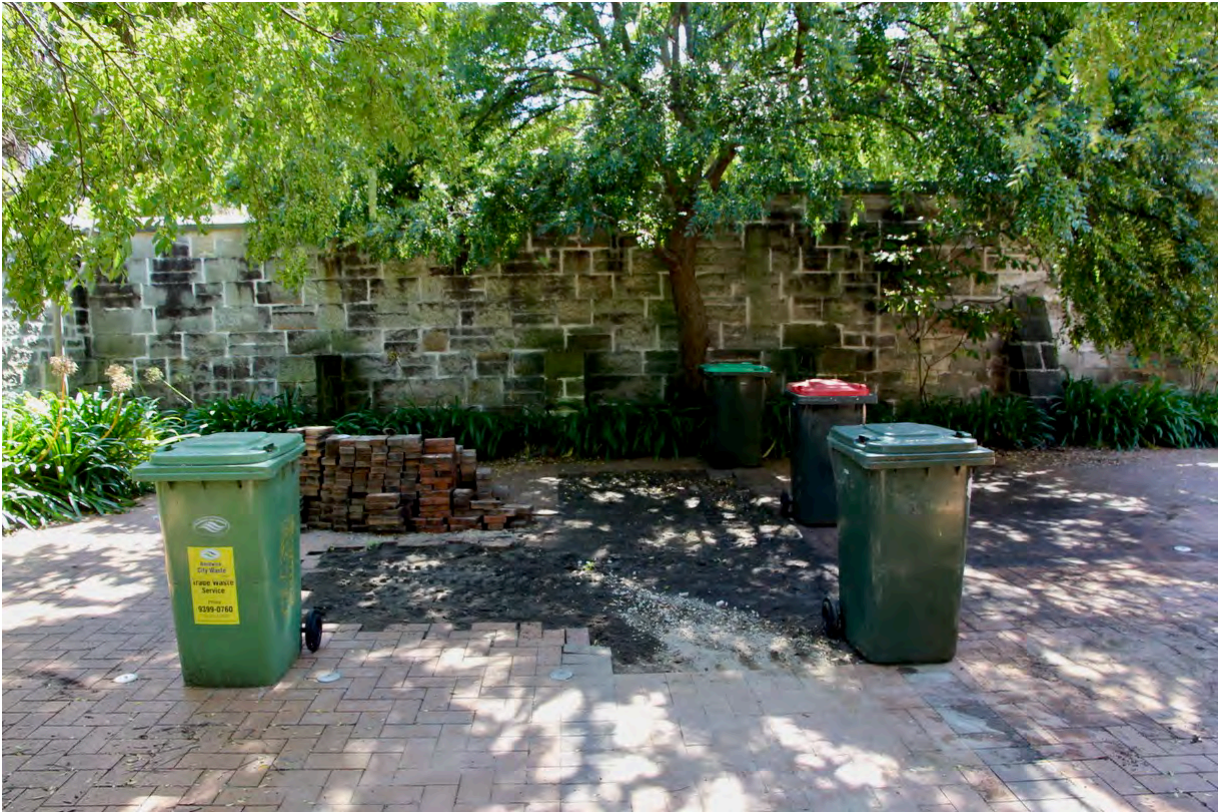
Figure 79: TT - After backfilling
