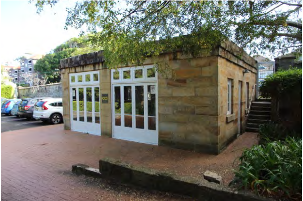
Figure 61: Cliffbrook (CC3 garage)
