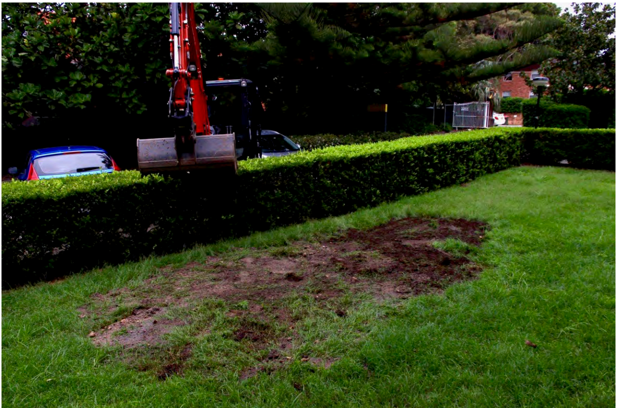
Figure 93: TT3 - After backfilling
