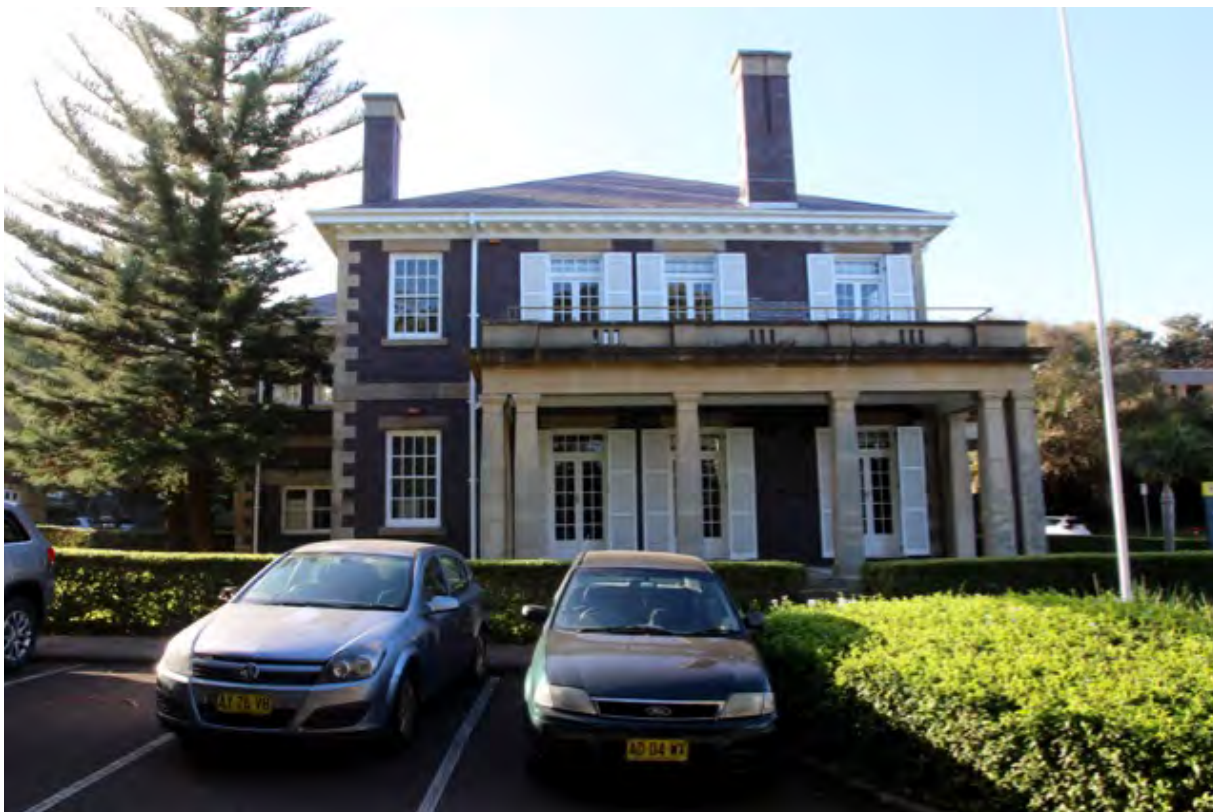
Figure 58: CliffBrook (souther facade & car parking)
