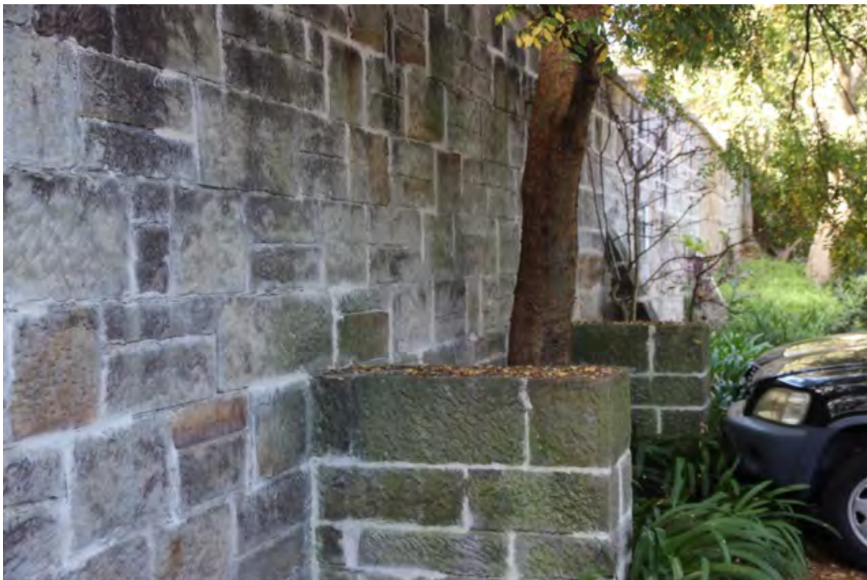
Figure 57: CliffBrook Campus (northern boundary wall buttressing)
