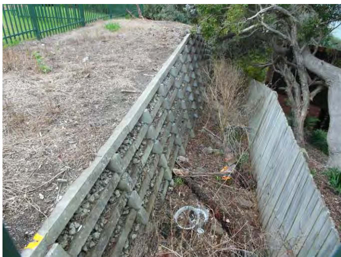
Figure 12. View south-east over built up retaining wall containing piped drainage.
