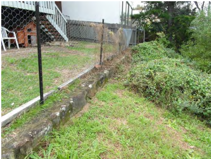
Figure 15. Property edging and footings are likely to have been carved from outcropping sandstone in the eastern third of the property.
