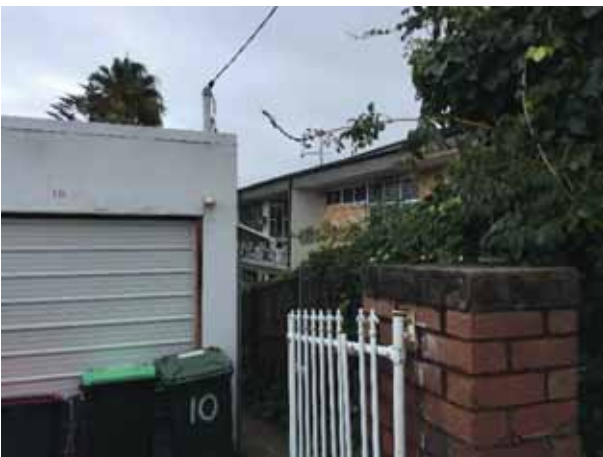
Picture 3 – Subject site from the Eastern Elevation (Battery Street)
