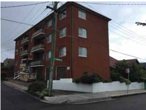
Picture 9 – Corner of Battery and Flood Streets
