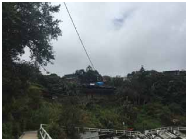
Picture 4 – Subject site from the Southern Elevation (Gordons Bay)
