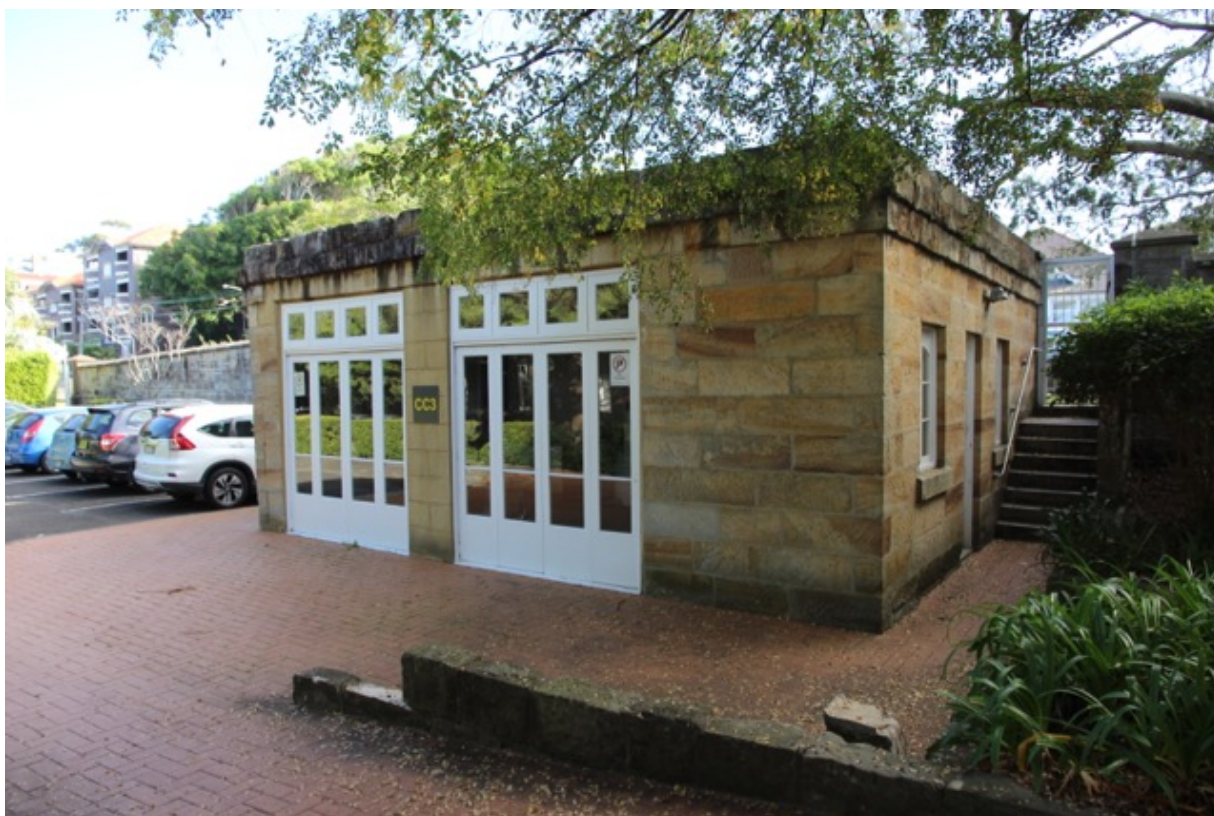
Figure 61: Cliffbrook (CC3 garage)
