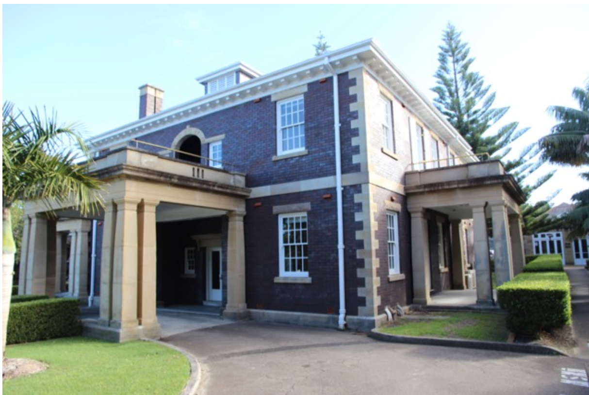
Figure 59: CliffBrook (eastern facade with stone portico)
