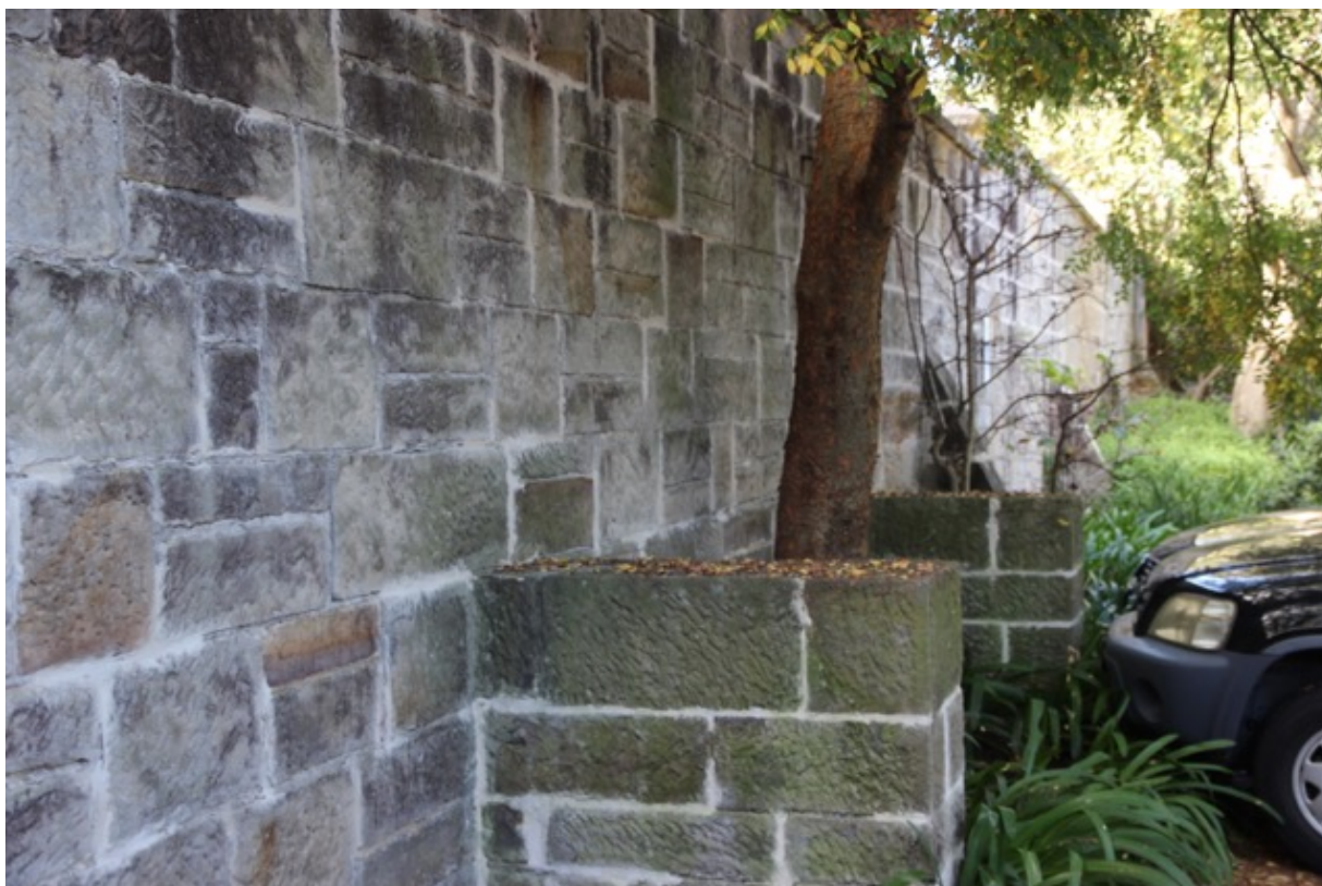
Figure 57: CliffBrook Campus (northern boundary wall buttressing)
